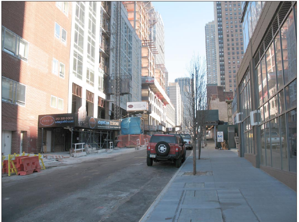
View of construction east on West 60th Street from West End Avenue 10
