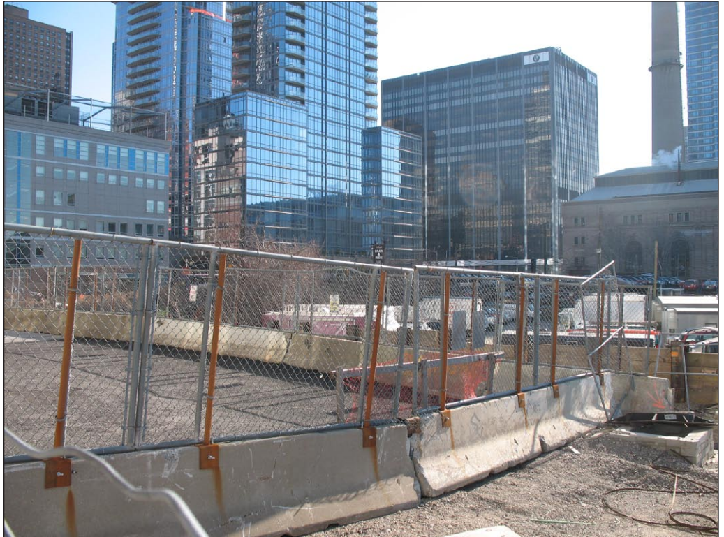
View southeast from project site to new development in study area 9
