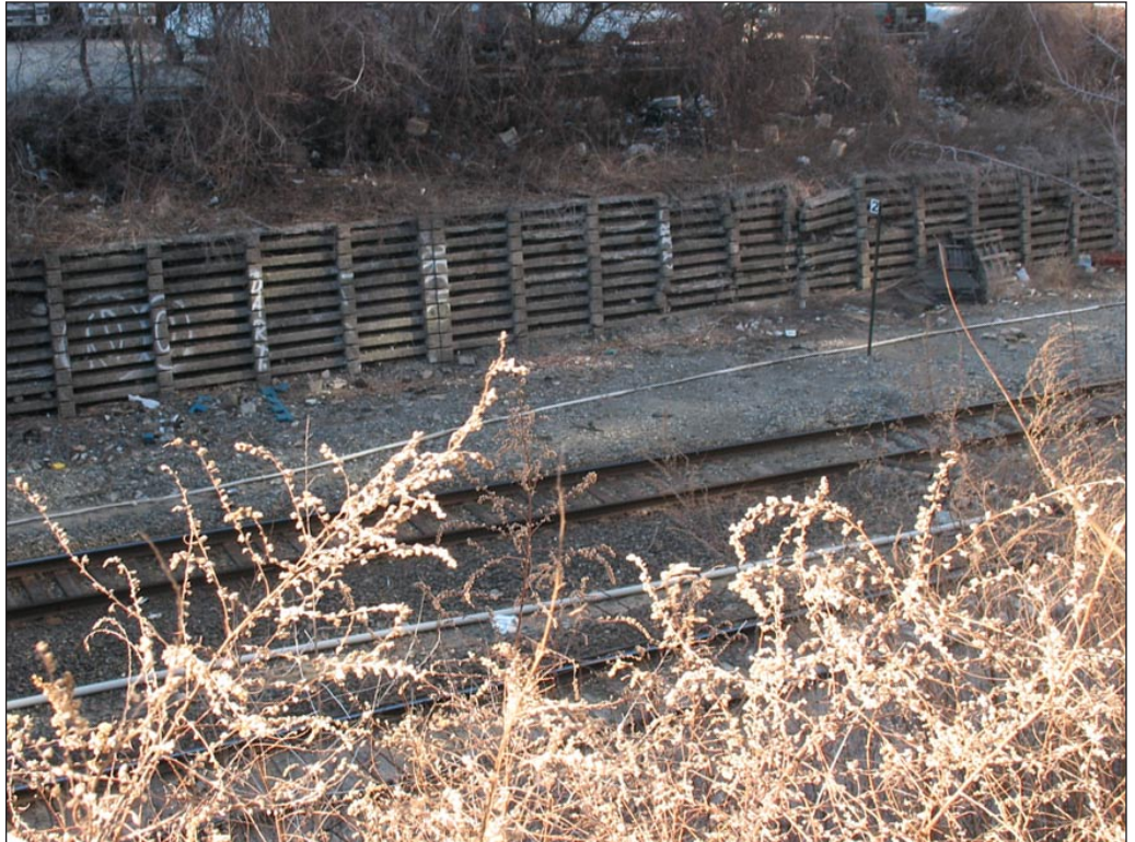
Amtrak culvert on project site, view from West End Avenue 3
