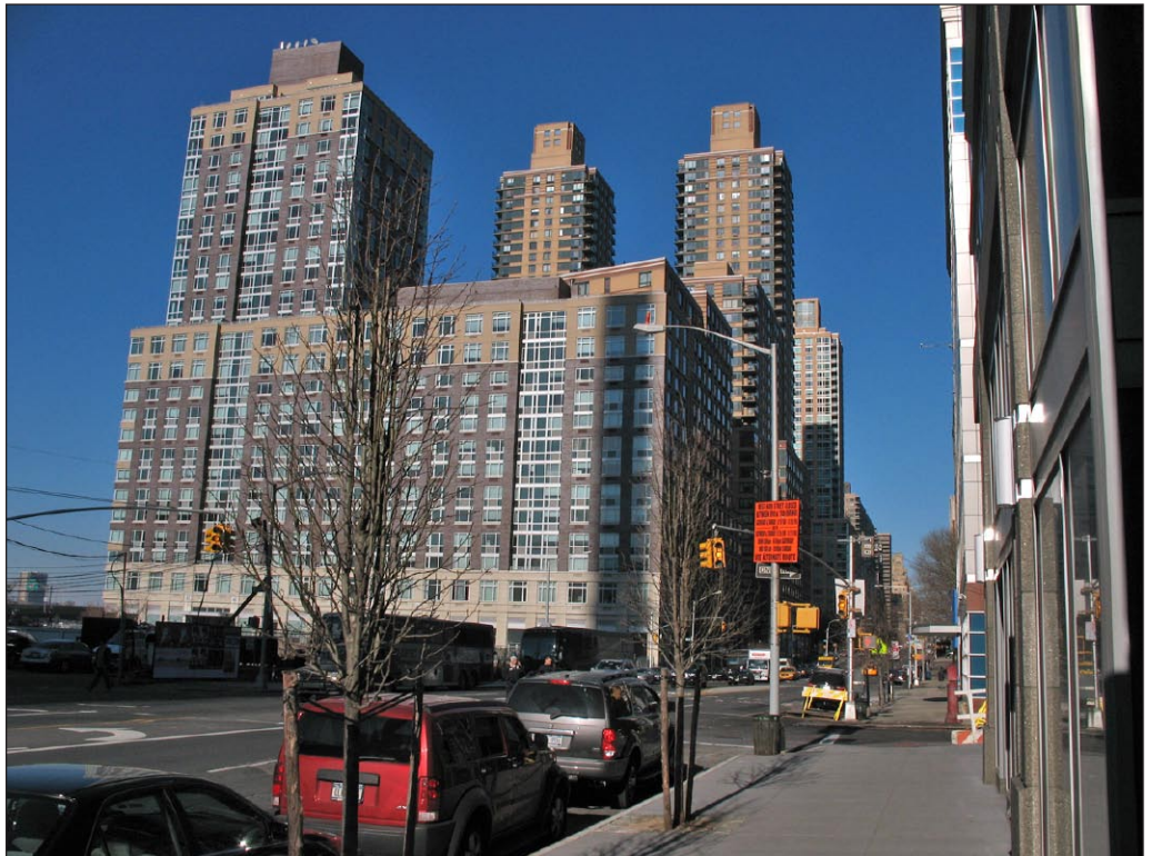
View north on West End Avenue toward Parcel O development 4
