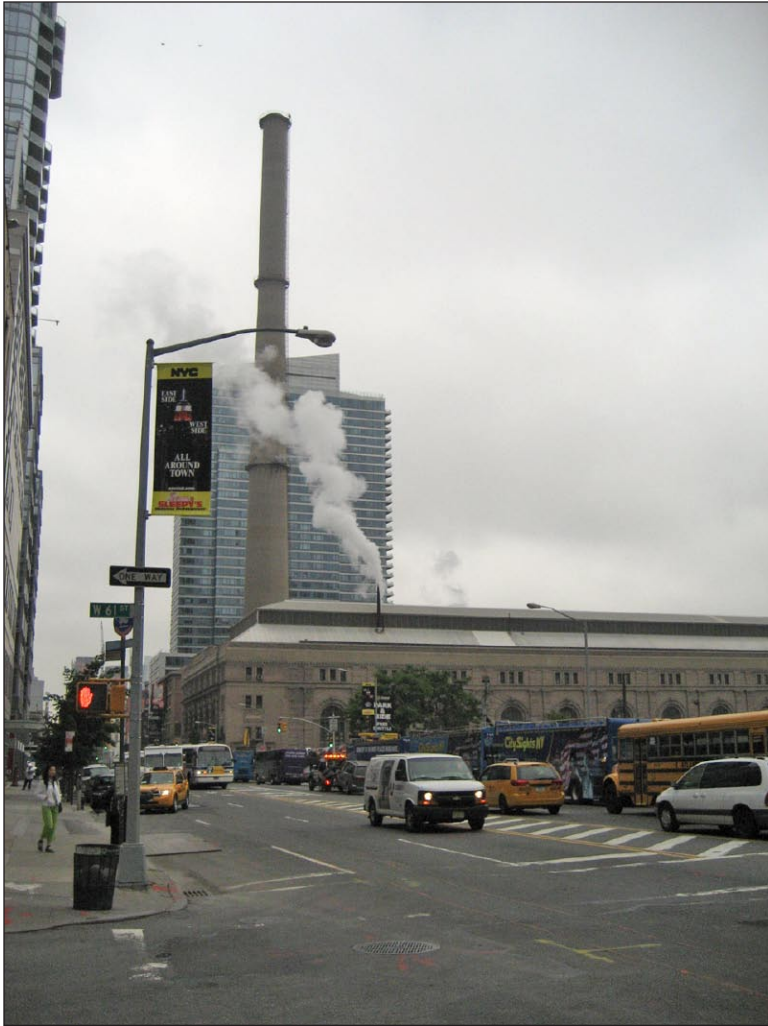
View south on West End Avenue to Consolidated Edison Power House 15
