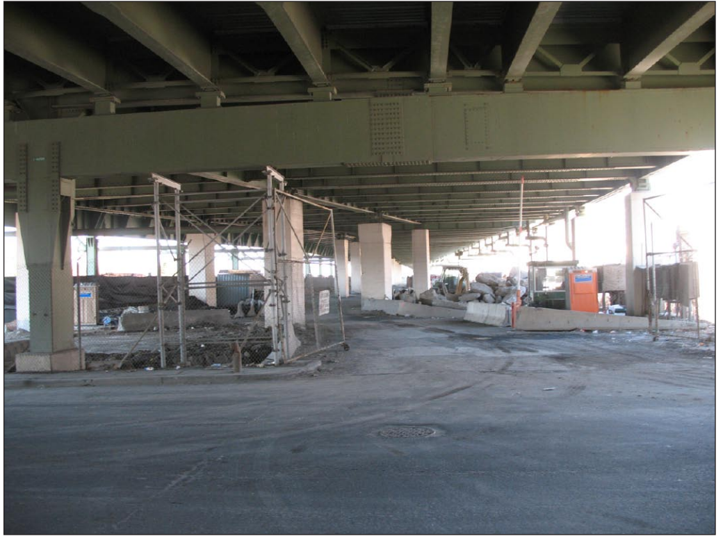
View north from West 59th Street, beneath Route 9A viaduct 13
