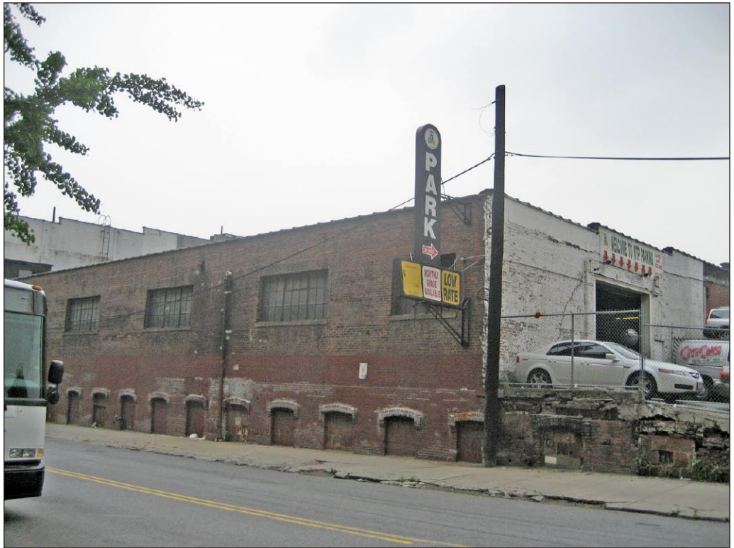
Two-story building on the project site, view northwest on West 59th Street
