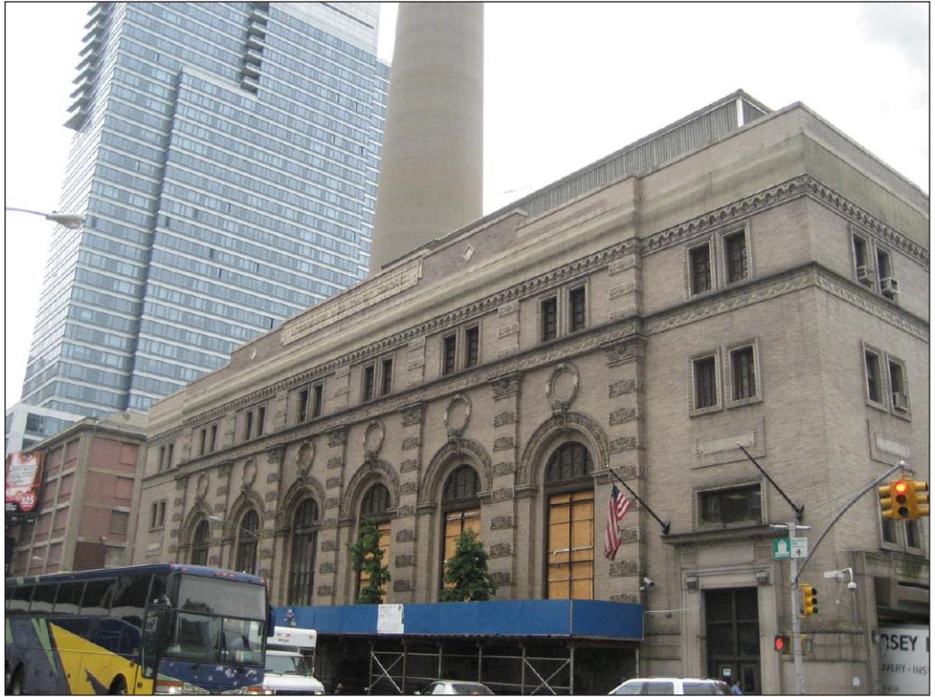
Consolidated Edison Power House, view southwest on West End Avenue 1
