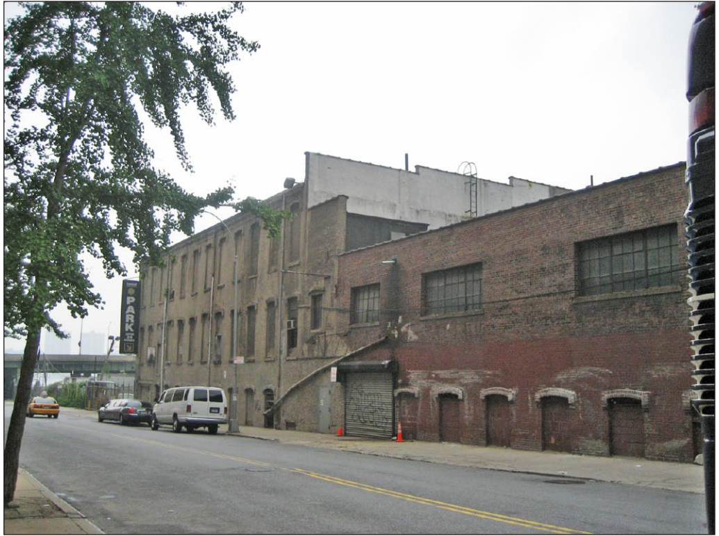
Three- and two-story buildings on the project site, view northwest on West 59th Street
