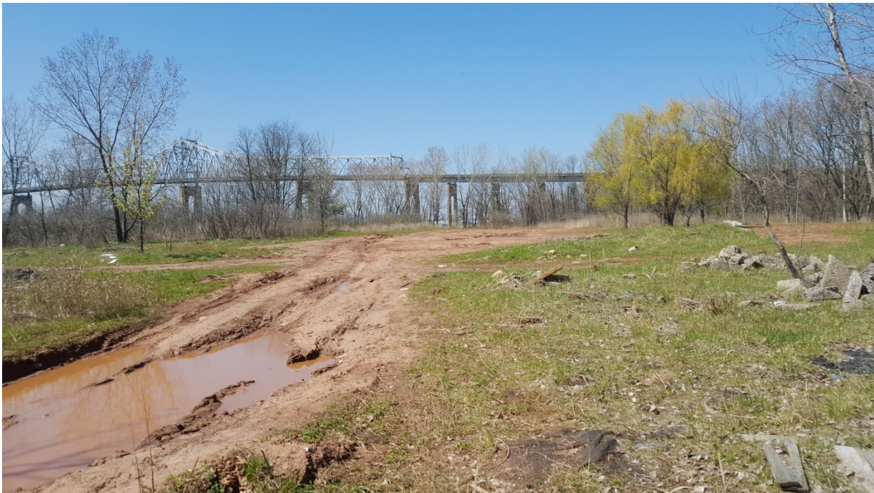
20 – South Center – View NW
