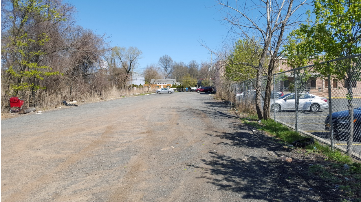
13 – North Roadway – View E
