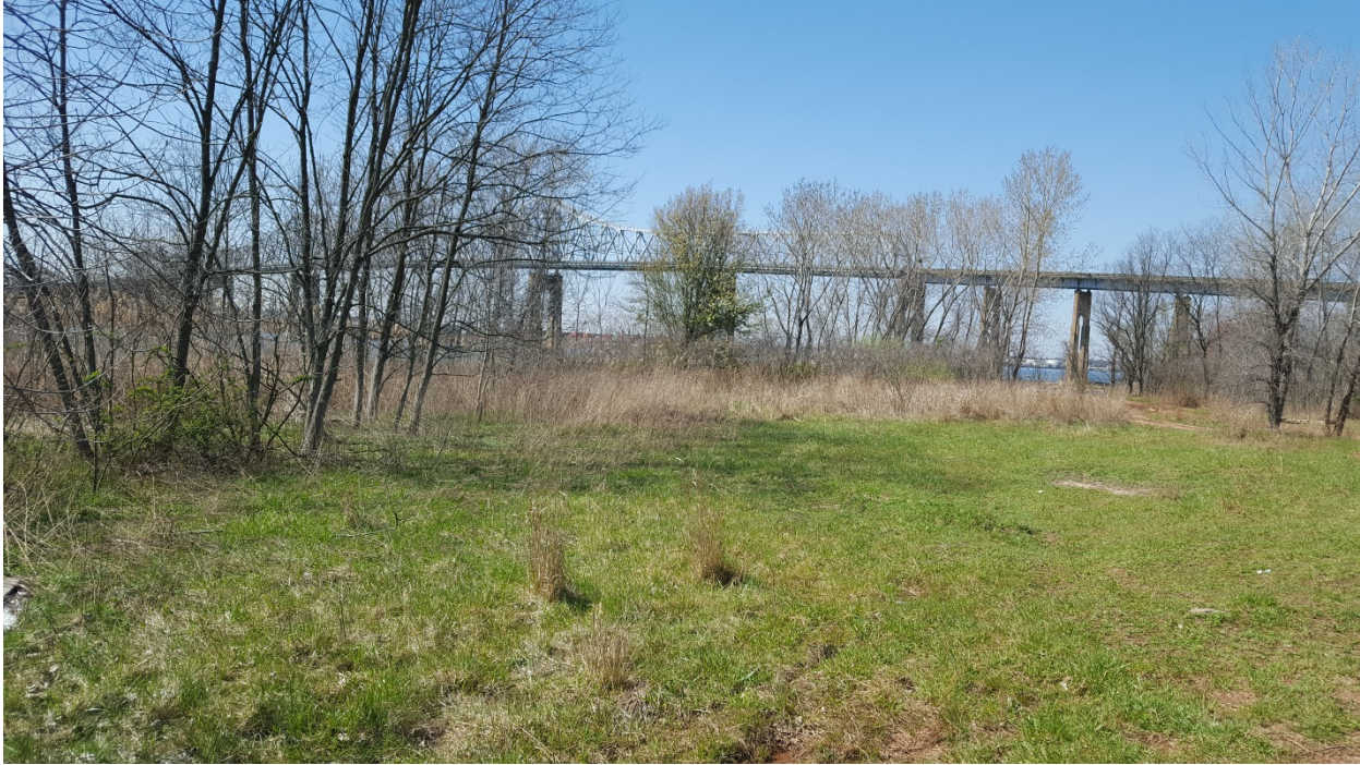
18 – South Center – View NW
