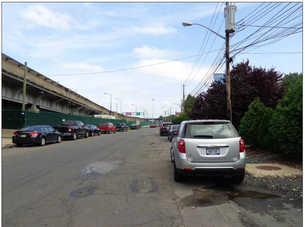
View east of the elevated ramp of the Outerbridge Crossing on South Bridge Street 4
