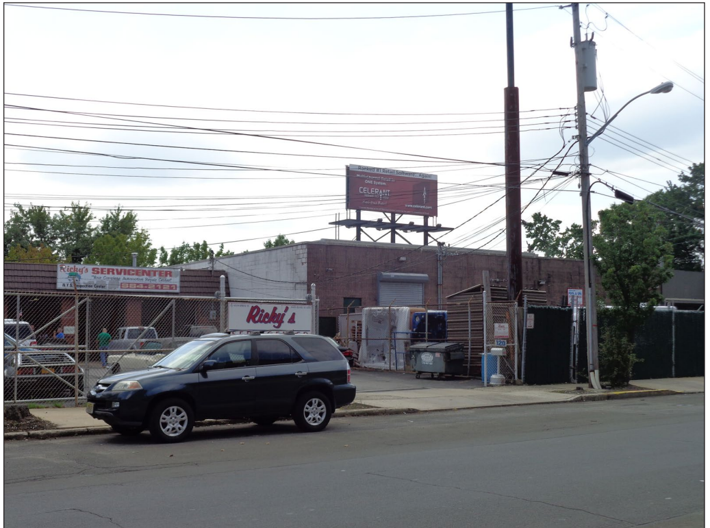
View southwest of the buildings on South Bridge Street 3
