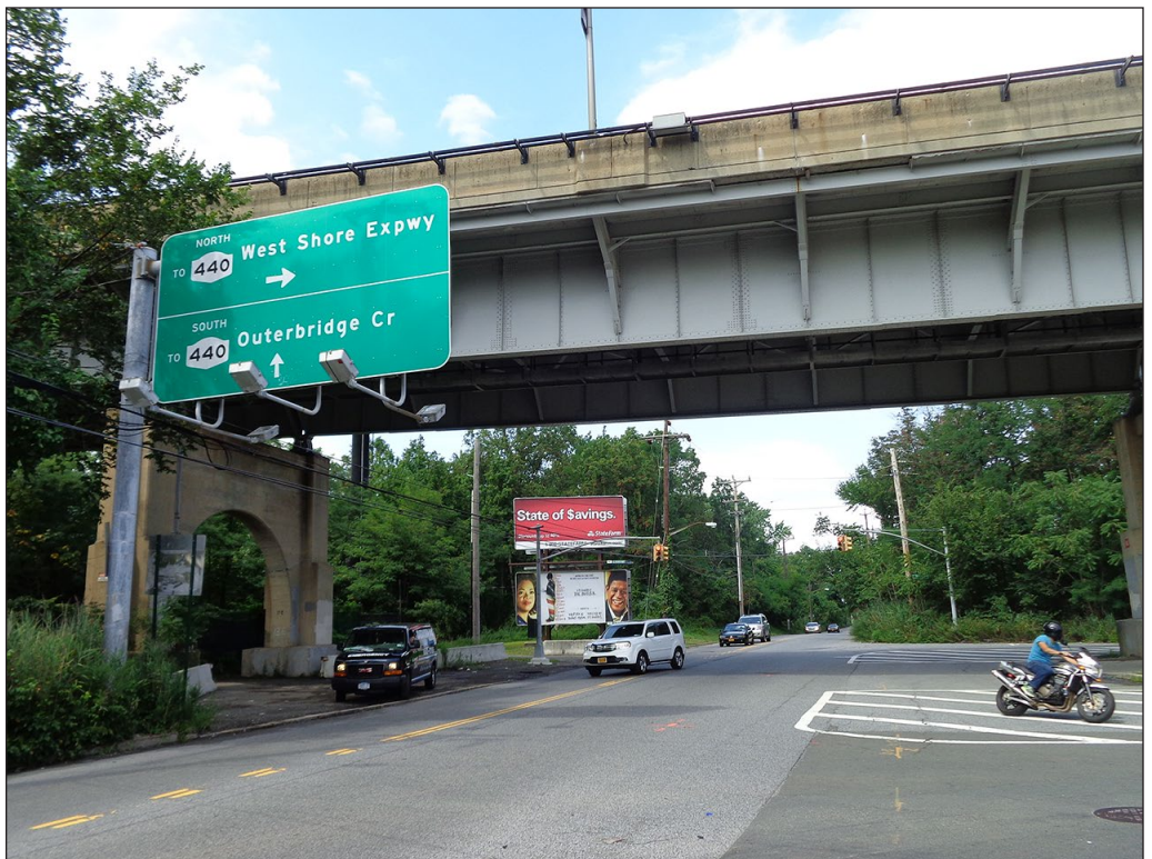
Outerbridge Crossing and transportation signage, view north from Arthur Kill Road 12
