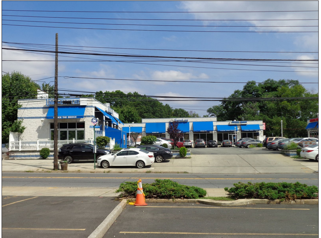
View east of the small shopping center on Arthur Kill Road 7
