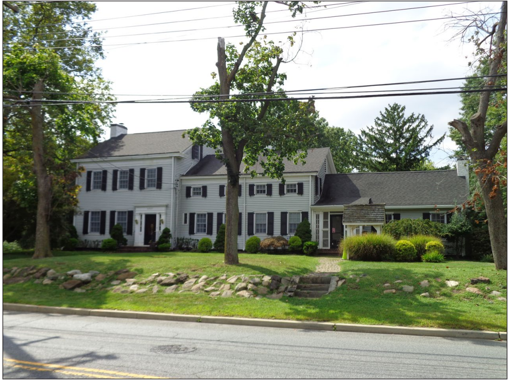
View west of the east façade of the Captain Abram and Ann Dissosway Cole House located at 4927 Arthur Kill Road
