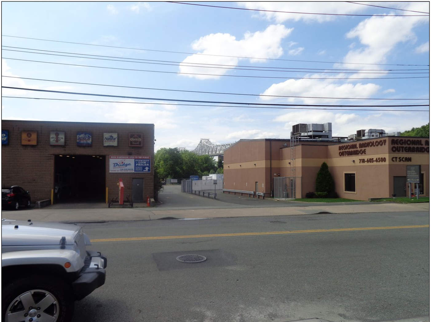
View west of the easternmost portion of the truss of the Outerbridge Crossing from Arthur Kill Road 3
