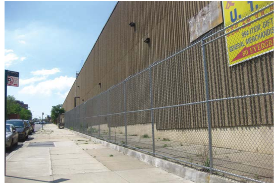
12. Block 3140- Facing southeast on Evergreen and Flushing avenues
