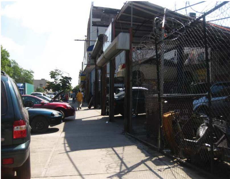
3. Block 3138-Facing northeast on Flushing Ave and Garden Street
