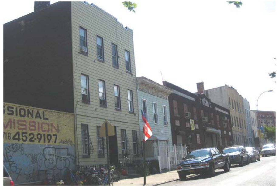
6. Block 3138- Facing southeast on Garden Street from Flushing Ave
