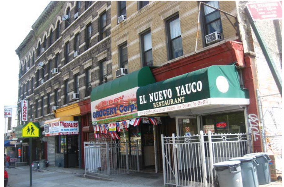
10. Block 3139- Facing north on Bushwick Ave and Montieth Street
