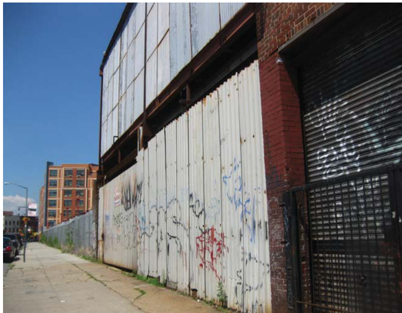
19. Block 3152- Facing southwest on Melrose Street mid-block
