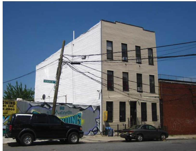
18. Block 3152- Looking west on Evergreen Ave and George Street
