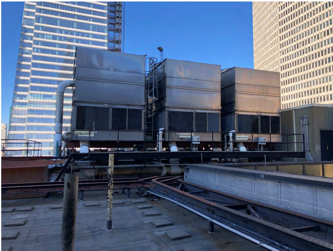
Photograph 19: Cooling towers located on the roof level.
