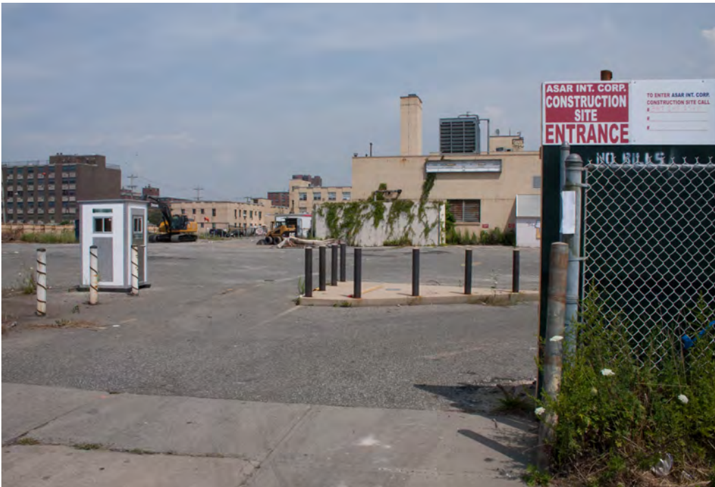
Photograph 6: View into Project Site, midblock, along Rockaway Beach Blvd.
