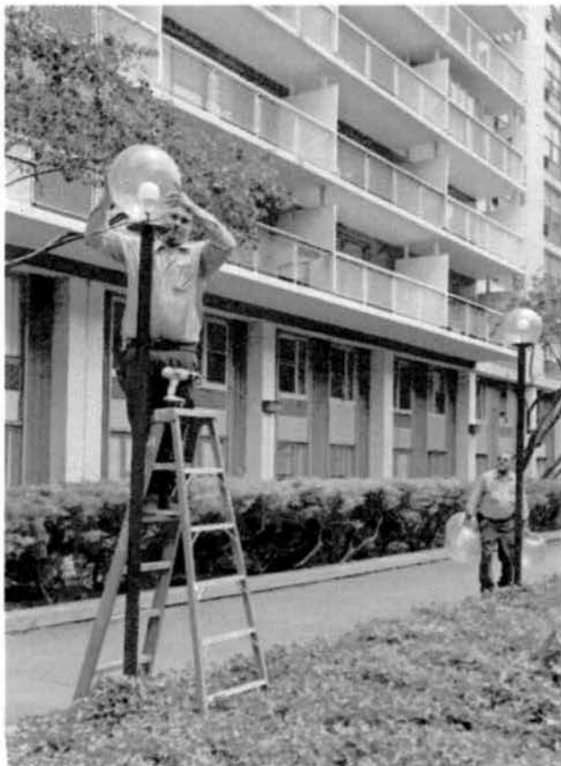
Cleaning Light Fixtures
