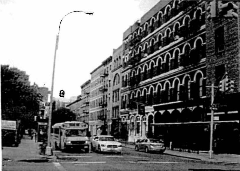
Figure 4 Buildings located along the western side of LaGuardia Place, across from proposed Blecker Building.
