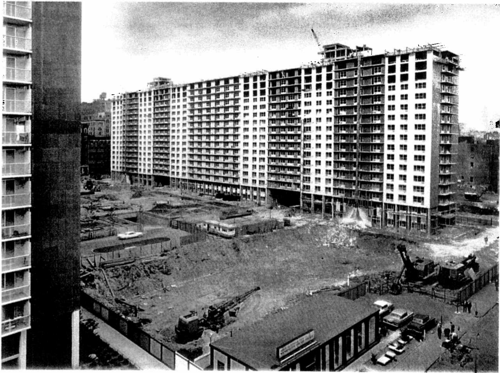
Washington Square Village under construction.. Wiener Collection, University of Oregon Library.
