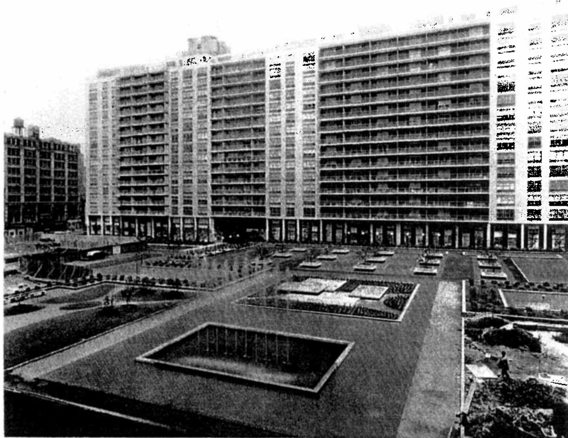
The garden under construction. Wiener Collection, University of Oregon Library.
