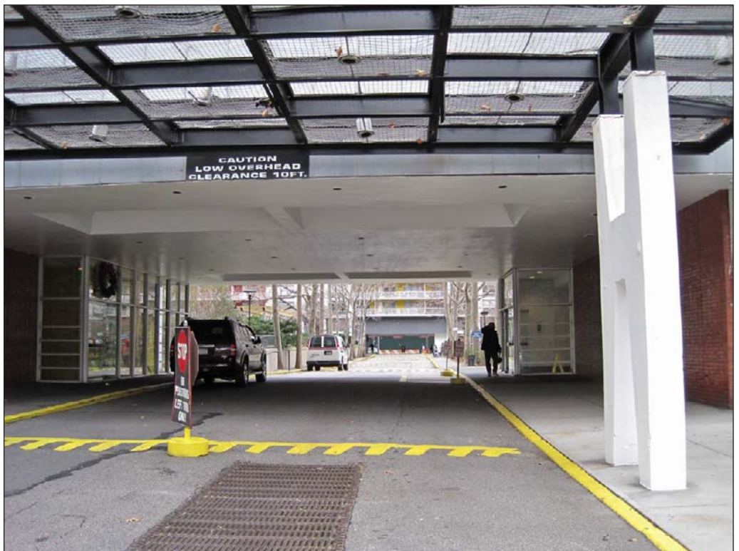
Washington Square Village, view north from Bleecker Street along east driveway 18
