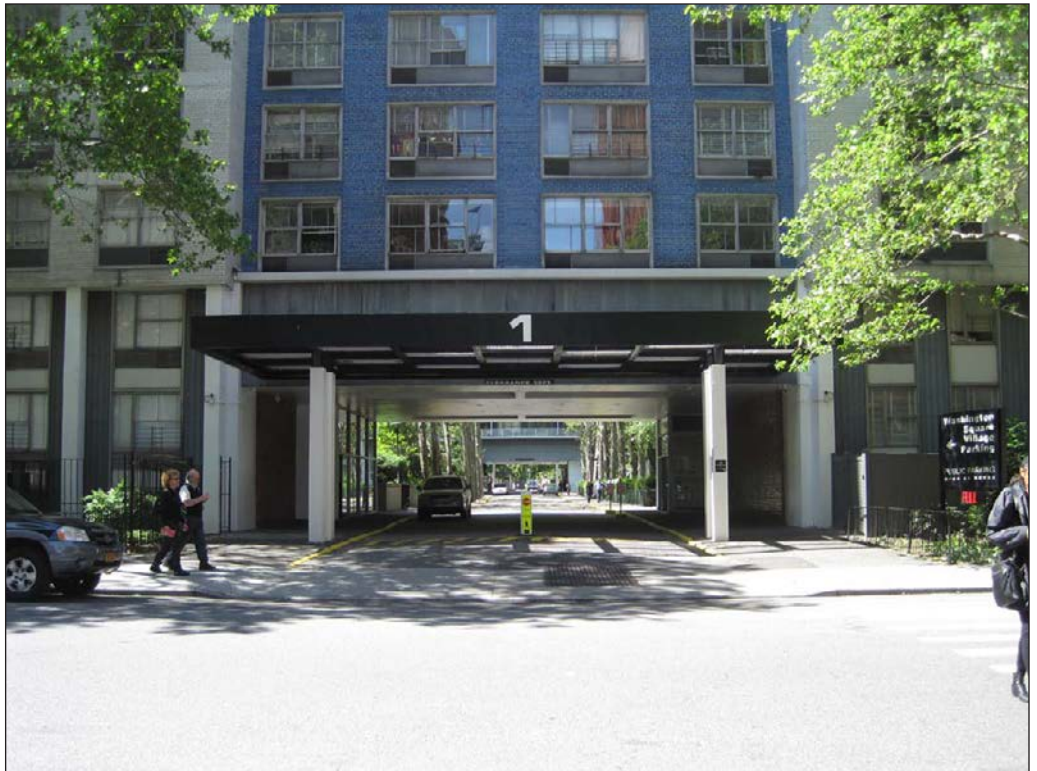
View south from West 3rd Street through the Washington Square Village northwest portal along the western driveway 86
