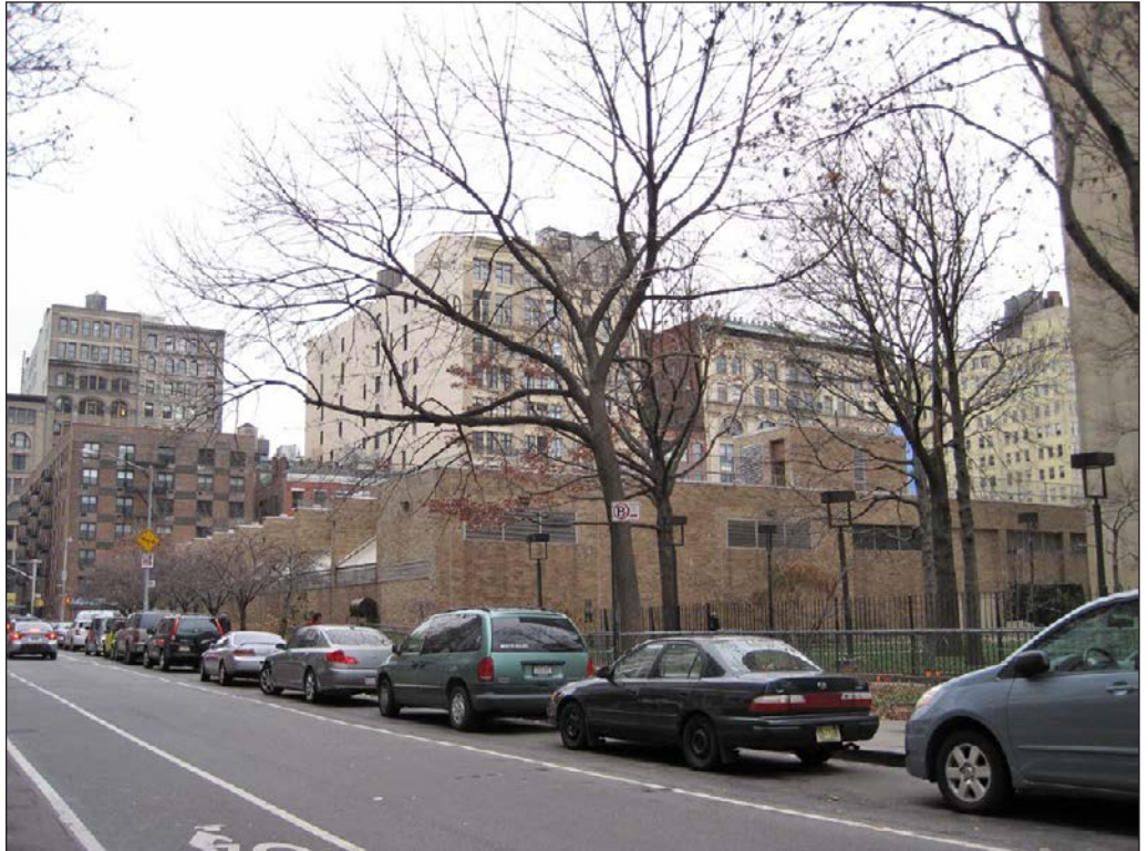
Coles Building, view southeast on Bleeker Street 11
