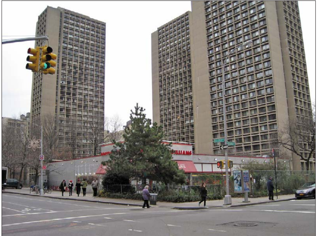
Grocery Store, view southeast from LaGuardia Place at Bleecker Street 7
