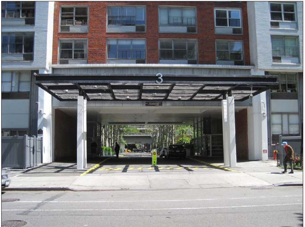
View north from Bleecker Street through the Washington Square Village southwest portal along the western driveway 88
