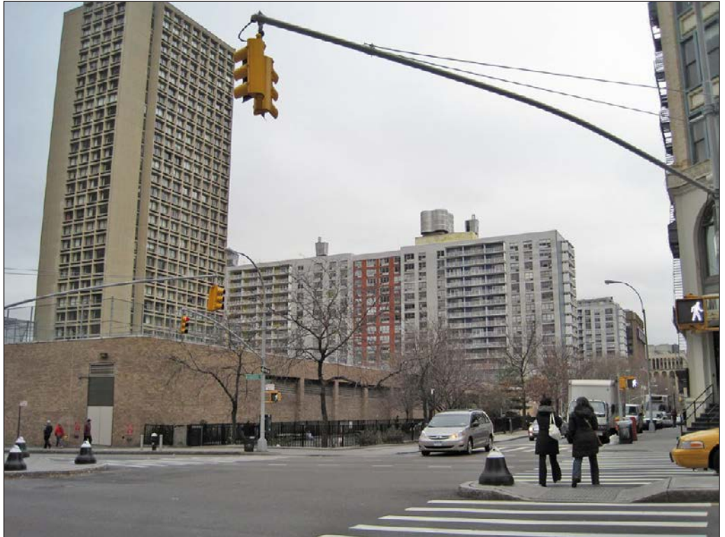
Coles Building, view northwest on Mercer Street from Houston Street 9
