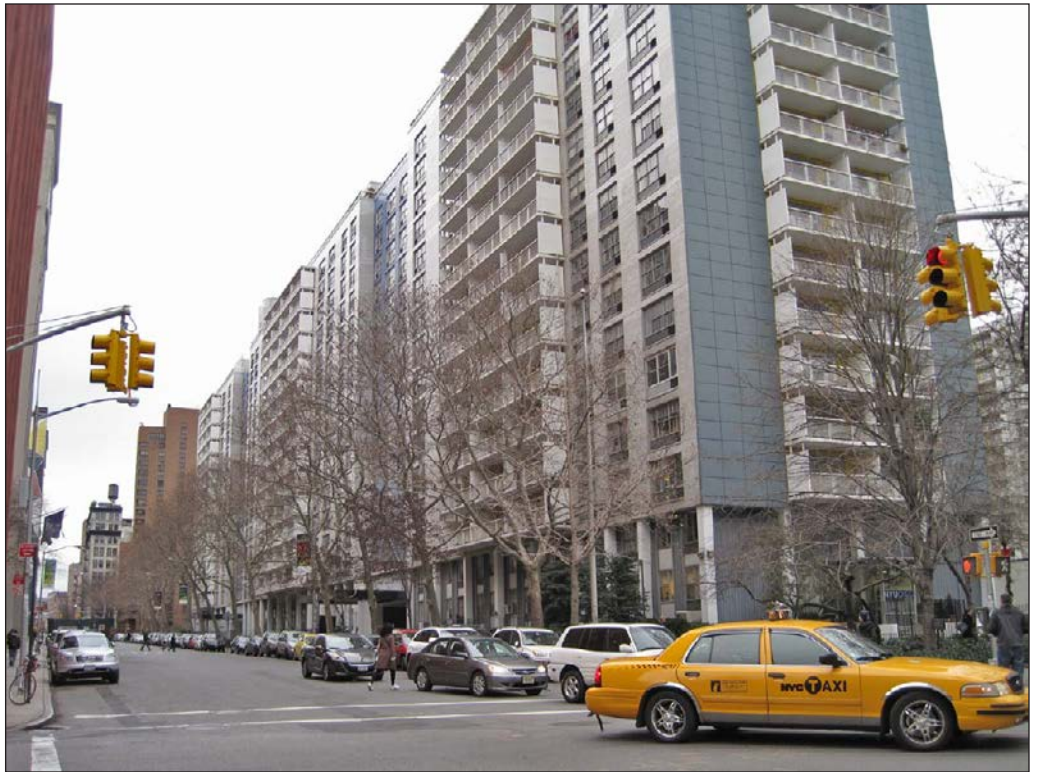
Washington Square Village, view east on West 3rd Street from LaGuardia Place 16
