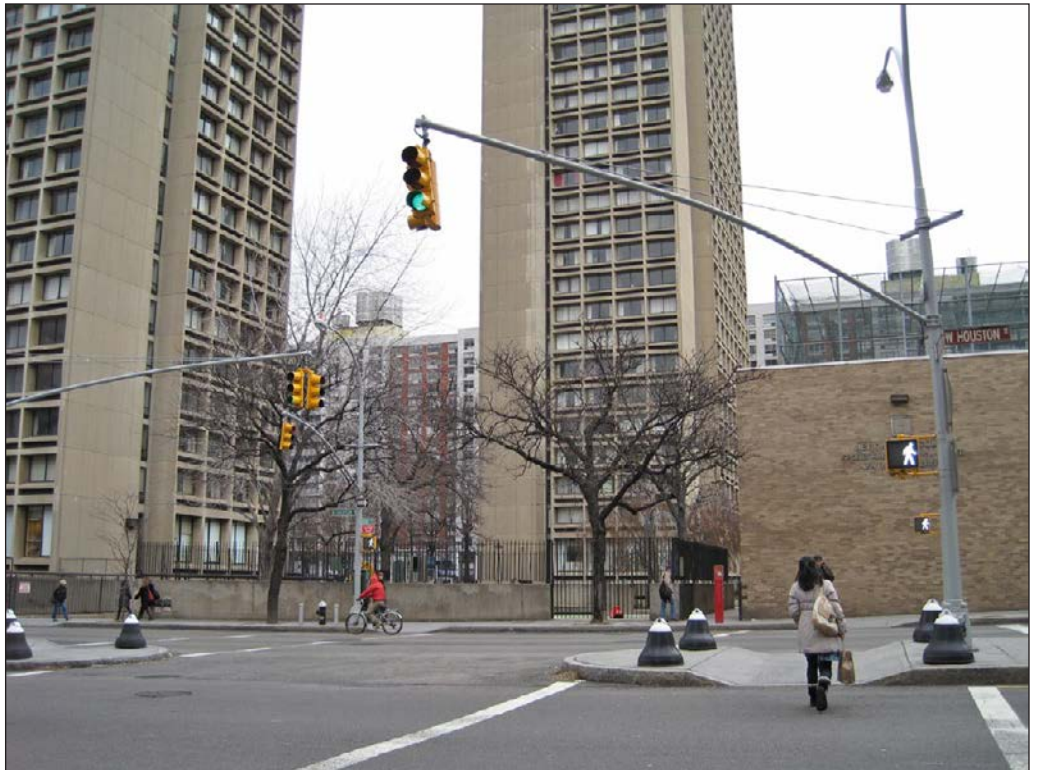
University Village, view north from Houston Street at Greene Street 4
