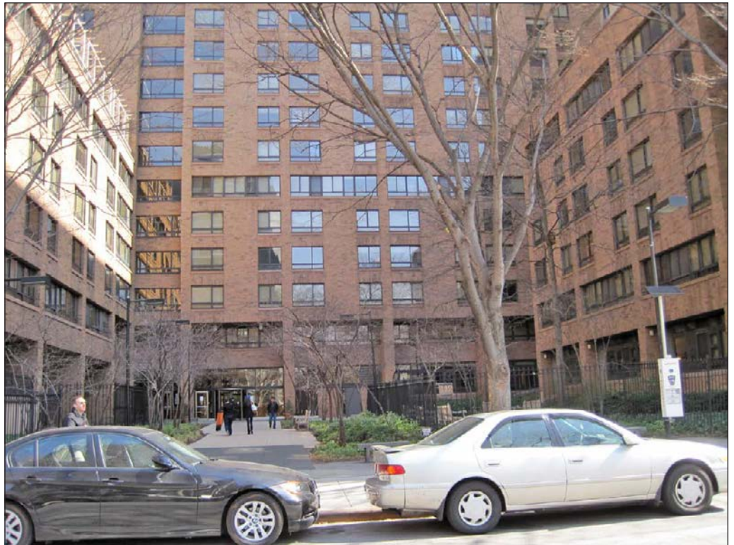
NYU Law School building, view east of courtyard from Mercer Street 56
