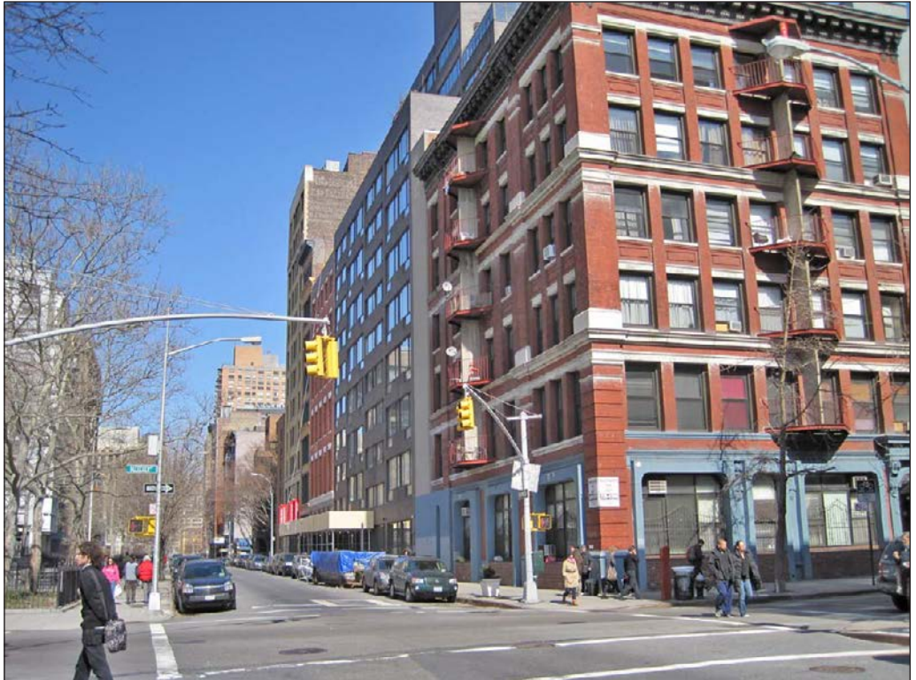
View northeast on Mercer Street from Blecker Street 60
