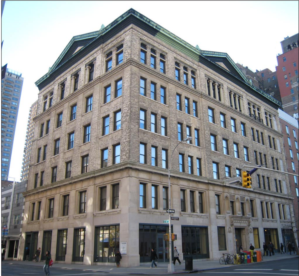
13-19 University Place/32-34 East 8th Street—North and west facades 27
