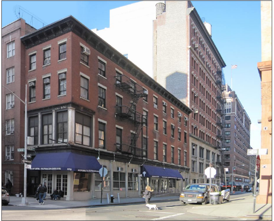
7 Washington Place/283 Mercer Street View E
