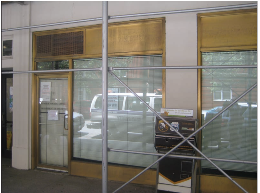
NYU Summer Housing Office (vacant), 14 Washington Place 4
