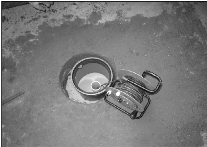
Photograph 3: Water level measurement collected at newly installed MW/CB-2.
