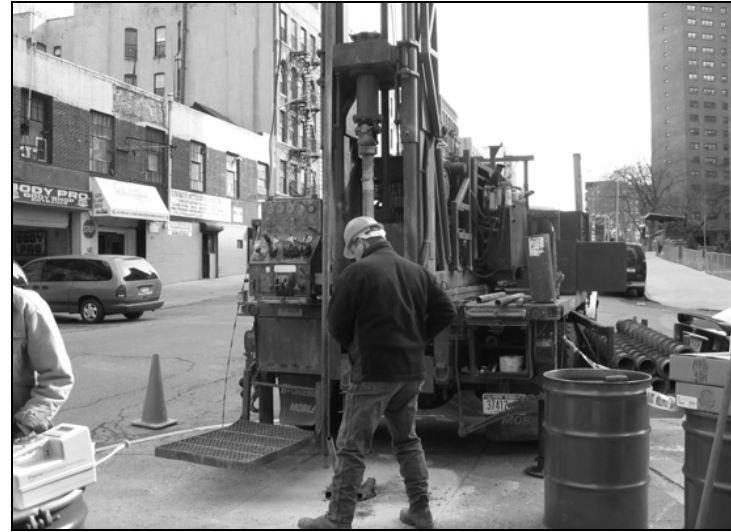
Photograph 2: Drilling activities at soil boring location MW/CB-1.
