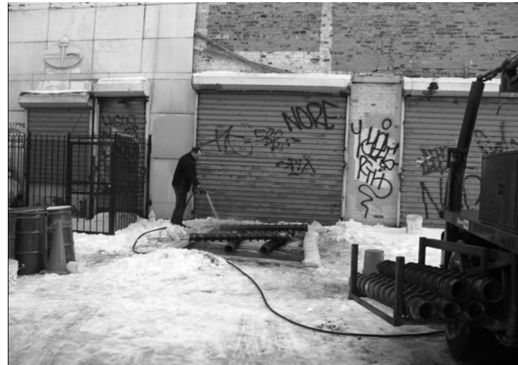
Photograph 4: Steam-cleaning the augers between soil boring locations.
