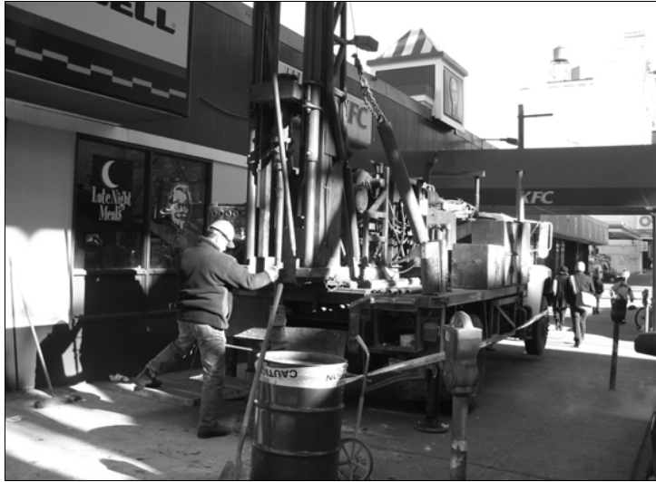
Photograph 1: Drilling activities at soil boring location MW/CB-20.
