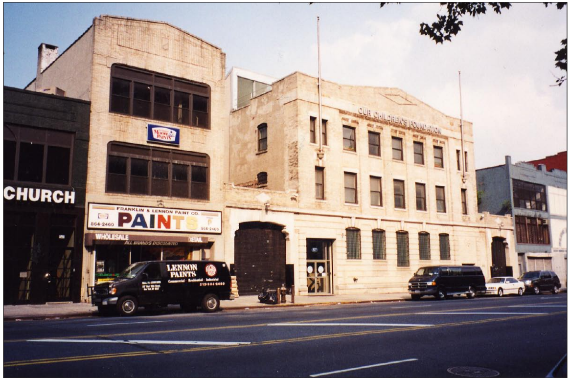
Former McDermott - Bunger Dairy, 527-535 West 125th Street 14
