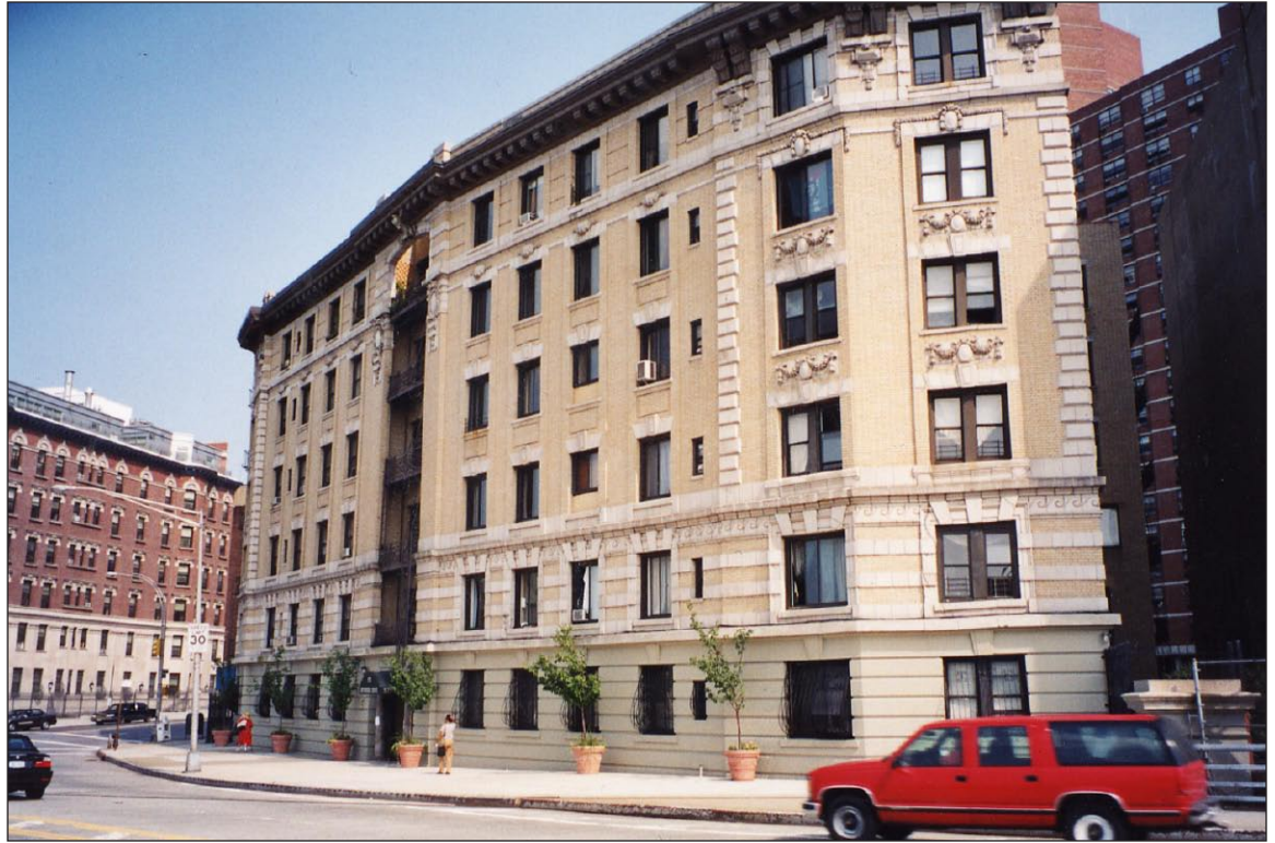
View of the southeast corner of Riverside Drive and West 135th Street (575 Riverside Drive)
