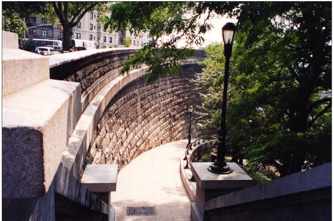
View south of Riverside Park stairs from Riverside Drive
