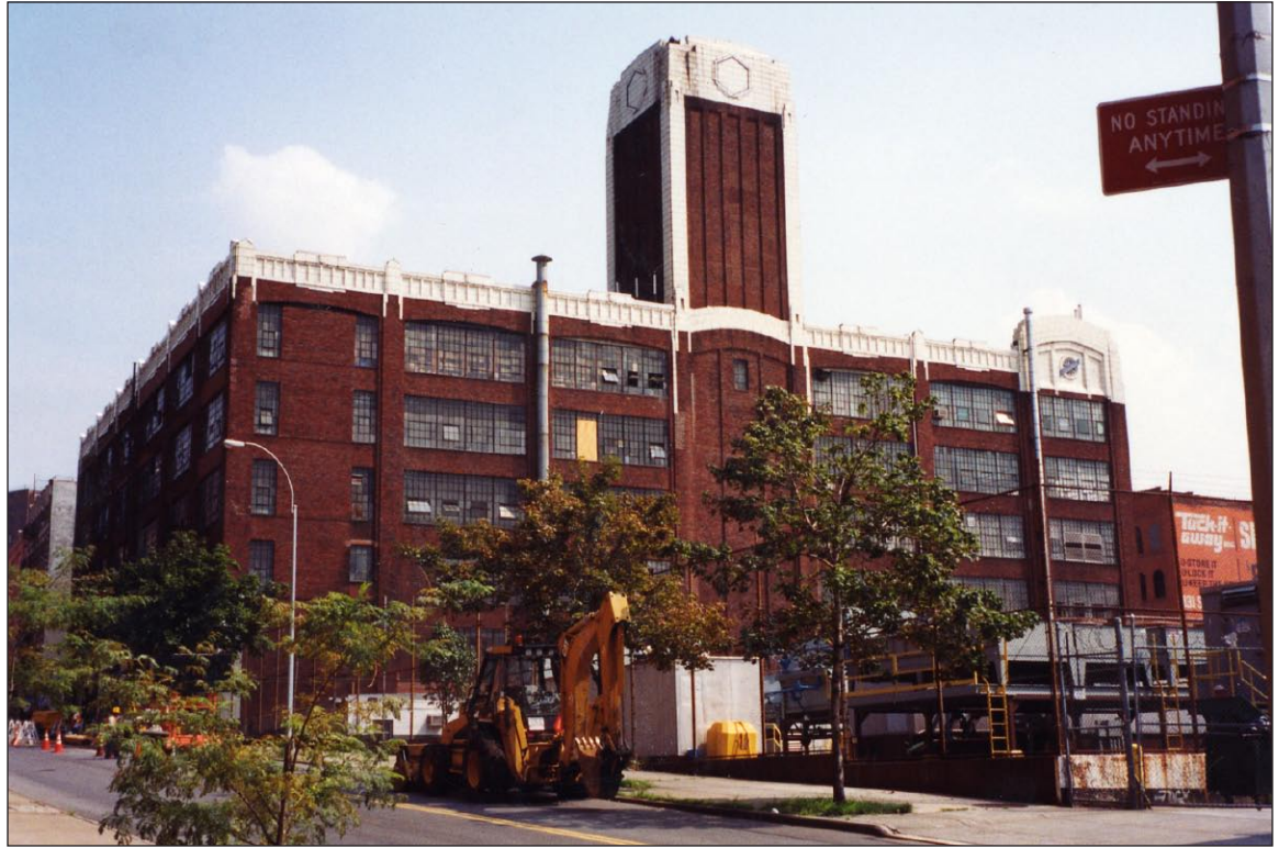
View southeast on West 132nd Street 3a
