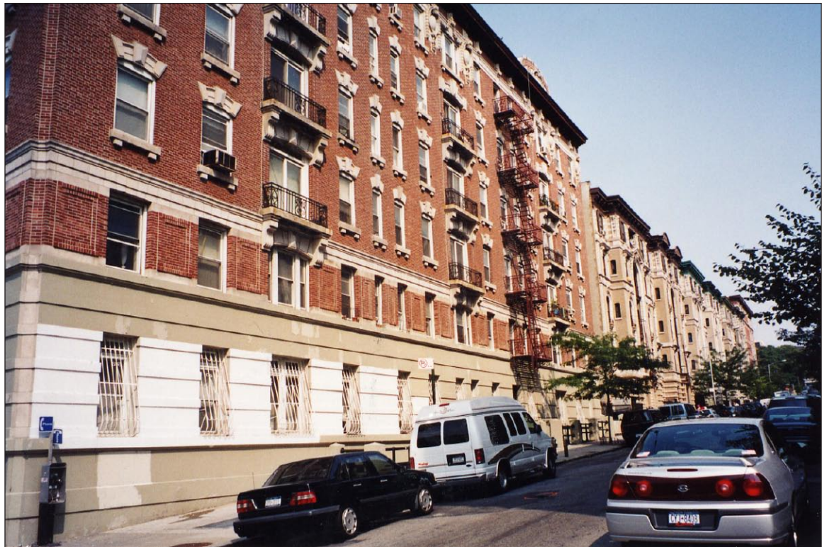
View from Riverside Drive of the north side of West 136th Street (590 Riverside Drive and 607-629 West 136th Street)
