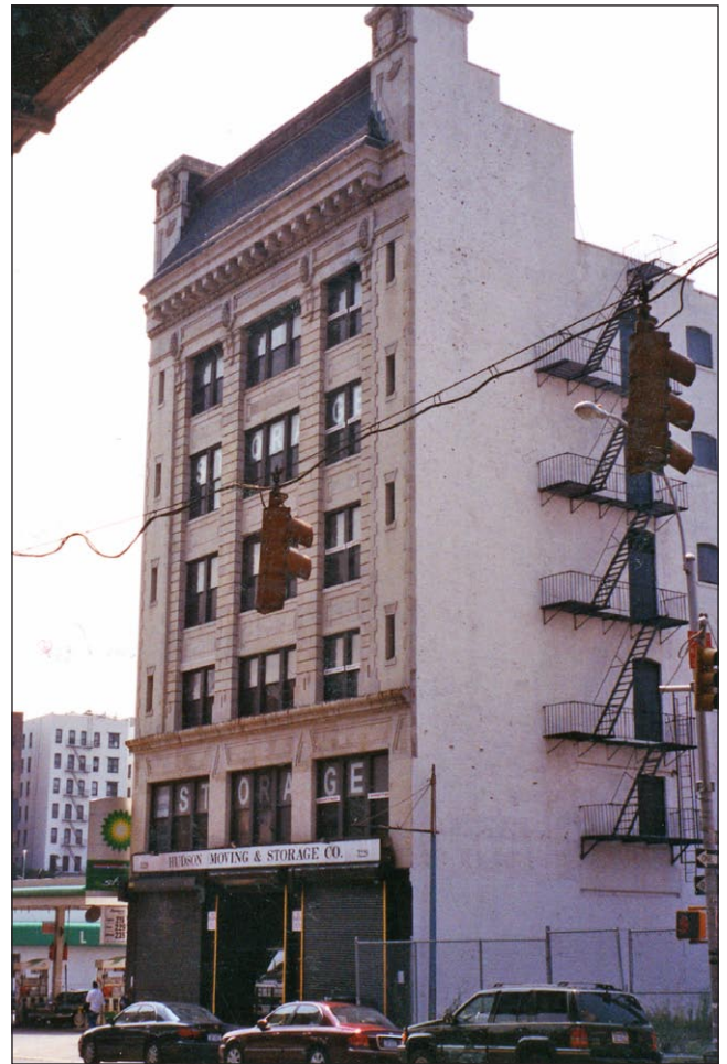
Former Stable, 3229 Broadway 5
