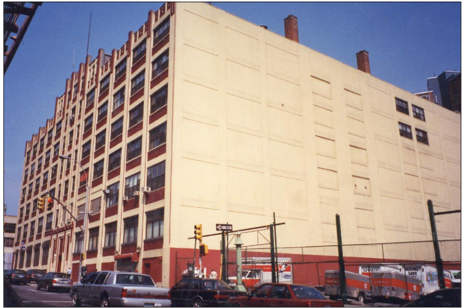
Former Warren Nash Service Center Building, 3280 Broadway 4
