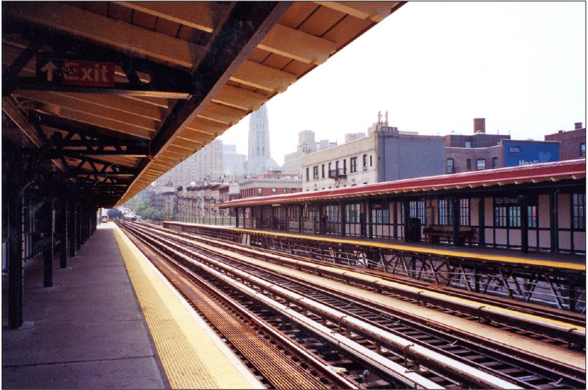
125th Street IRT Subway Station. View north at platform level 2
