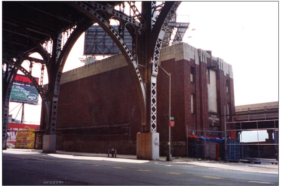
Former New York Central Railroad Substation No. 11, 2350-2362 Twelfth Avenue/ 700 West 134th Street 8
