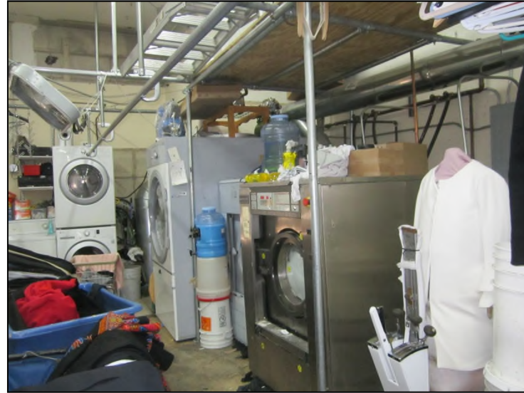
Photograph 26. Washing machines in the dry cleaner space.
