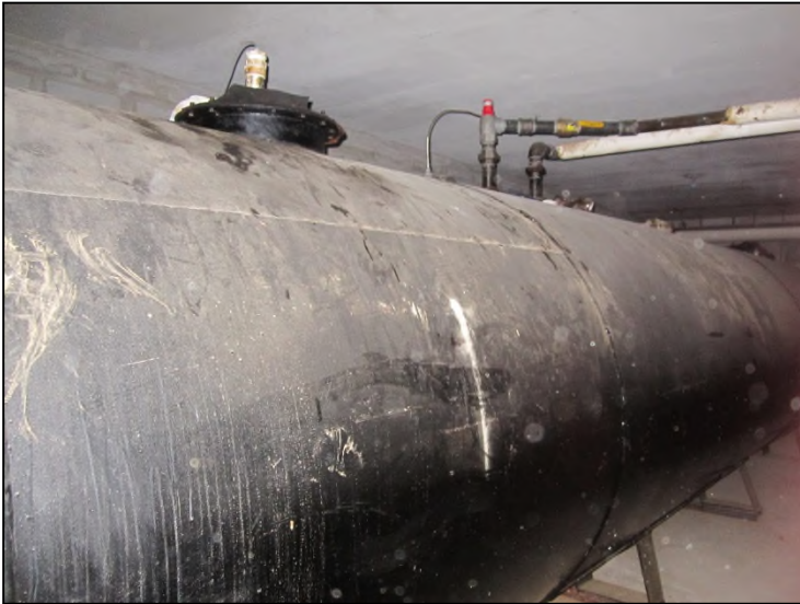
Photograph 9. A 10,000-gallon No. 4 fuel oil AST in the tank room of 45 West 132 nd Street.
