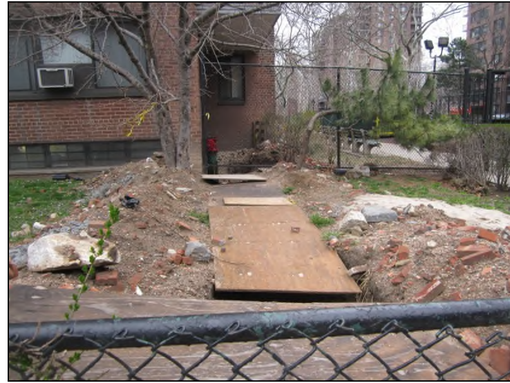
Photograph 10. A trench for future gas line installation on the eastern side of 45 West 132 nd Street, view north.
