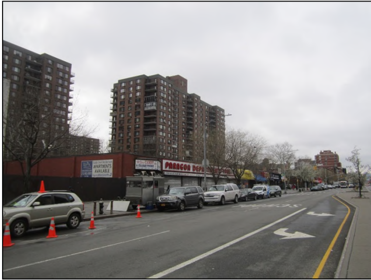
Photograph 17. The Property building on the southern side of Lot 68, view southeast.
