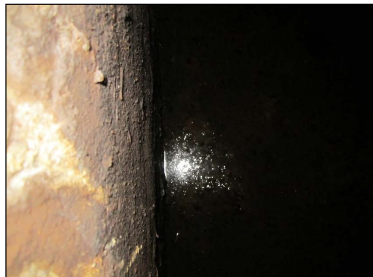
Photograph 4. Water with a slight sheen in the sump in the 470 Lenox Terrace boiler room.
