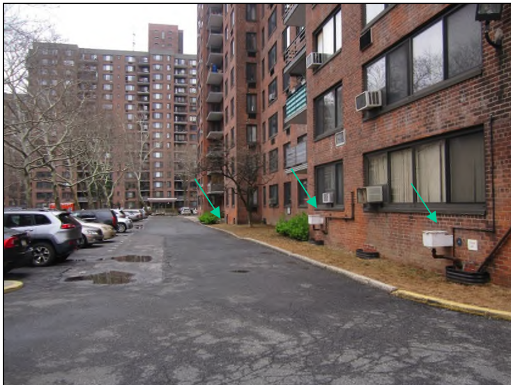
Photograph 7. Vent pipes and fill ports for two 10,000-gallon ASTs, and a vent pipe at the site of a closed-in-place 25,000-gallon UST, on the north side of the Property building at 45 West 132 nd Street, view east.
