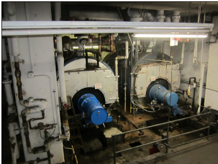
Photograph 11. Boilers in the basement of 25 West 132 nd Street.
