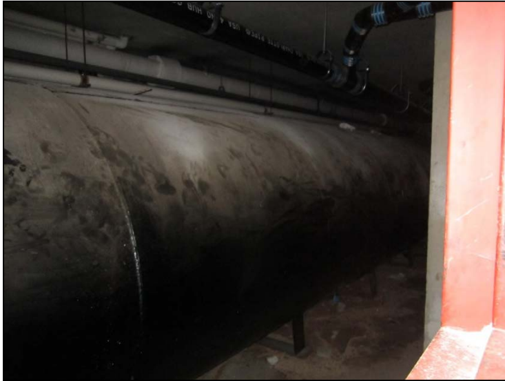
Photograph 5. A 10,000-gallon No. 4 fuel oil AST in the tank room of 470 Lenox Terrace.
