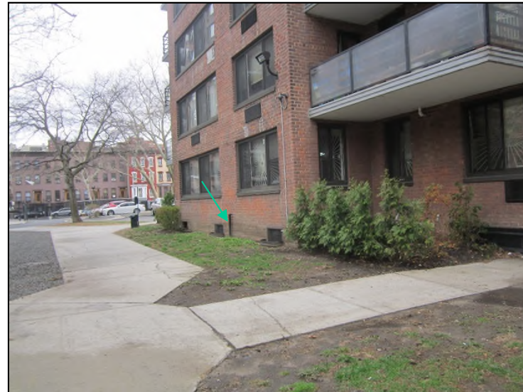
Photograph 6. A vent pipe at the location of a 25,000-gallon No. 6 fuel oil underground storage tank (UST) closed-in-place next to 470 Lenox Terrace.
