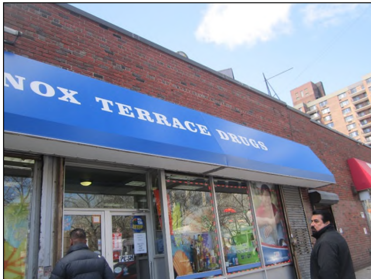
Photograph 23. The commercial Property building on Lots 50 and 52, view southwest.
