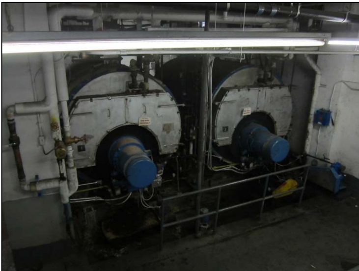
Photograph 3. Boilers in the basement of 470 Lenox Terrace.
