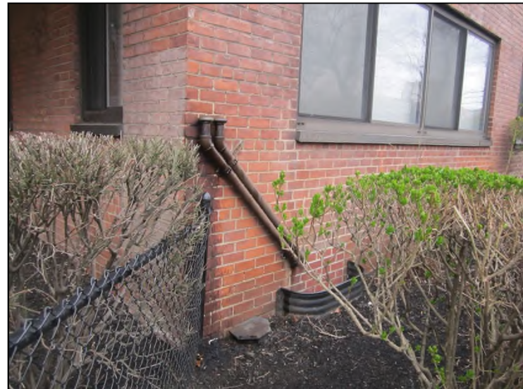
Photograph 2. Vent pipes for 10,000-gallon No. 4 fuel oil aboveground storage tanks (ASTs) on the façade of the Property building at 470 Lenox Terrace.
