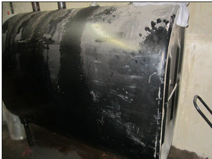
Photograph 27. An approximately 275-gallon No. 2 fuel oil AST with evidence of leakage in the basement of the dry cleaner.
