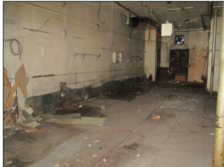
Photograph 20. A former dry cleaning space in the building on Lot 33.
