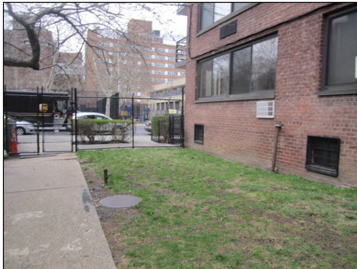
Photograph 15. A fill port, vent pipe and manhole (suspect UST access port) west-adjacent to the Property building at 10 West 135 th Street, view north.
