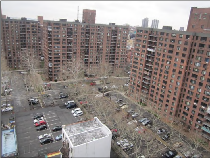
Photograph 1. Apartment buildings and parking on the Property, view southeast.
