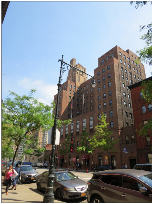
South side of West 135th Street, view from near Adam Clayton Powell Jr. Boulevard 16
