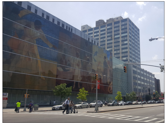
East side of Lenox Avenue, view from West 137th Street 18
