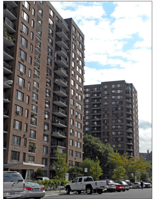
South side of proposed development site, view east near Lenox Avenue 6
