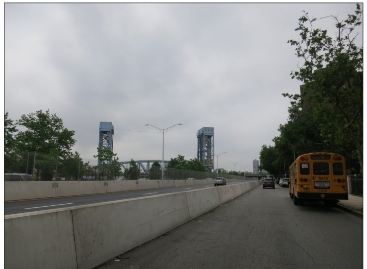
Harlem River Drive, view southeast from near 138th Street 15
