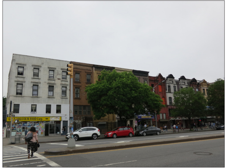
West side of Lenox Avenue, view from 132nd Street 22
