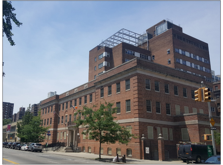
West side of Fifth Avenue, view from 137th Street 19
