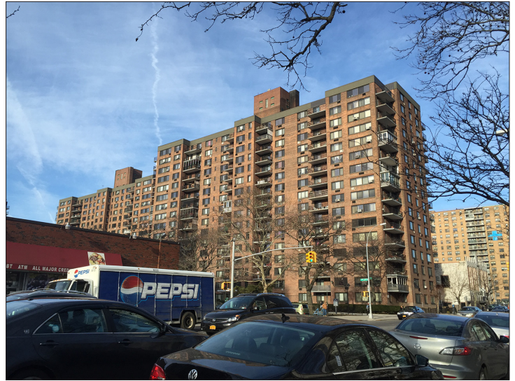
North side of proposed development site, view west from near Fifth Avenue 2
