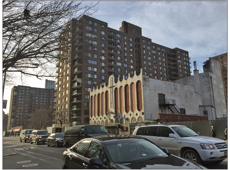
North side of proposed development site, view east from Lenox Avenue 1
