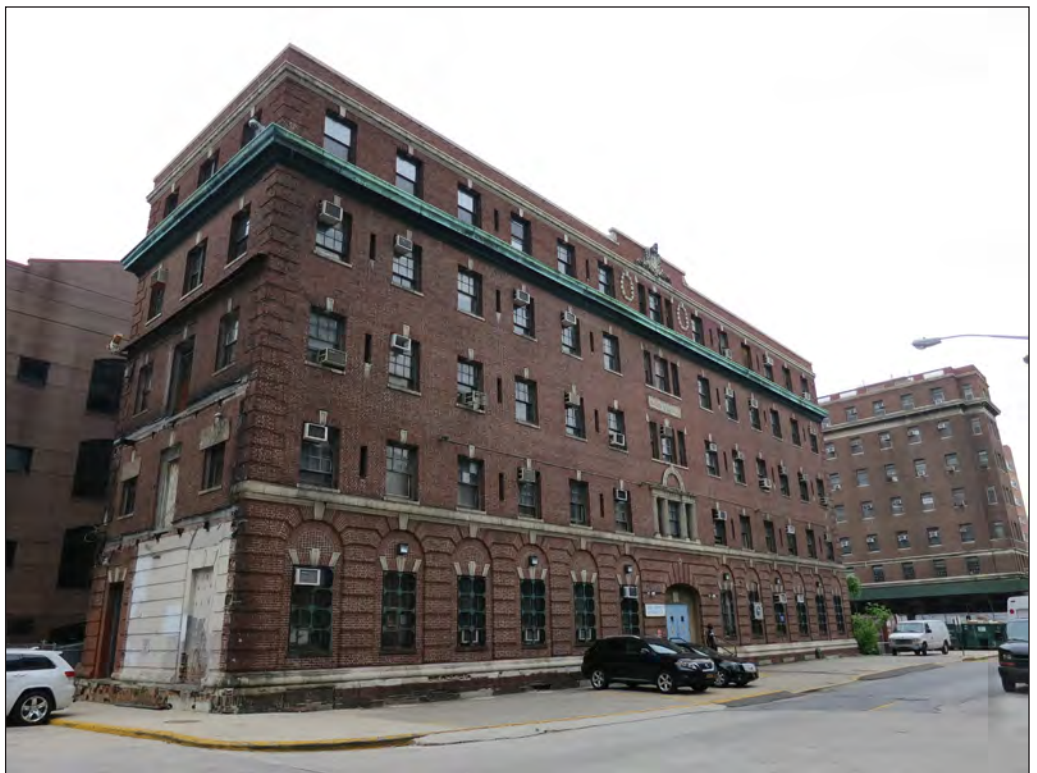
Harlem Hospital Center, Old Nurses Residence, view from 136th Street 12
