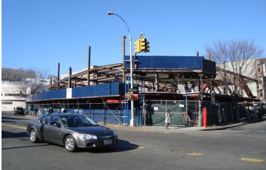
MHHC under construction (2009)
