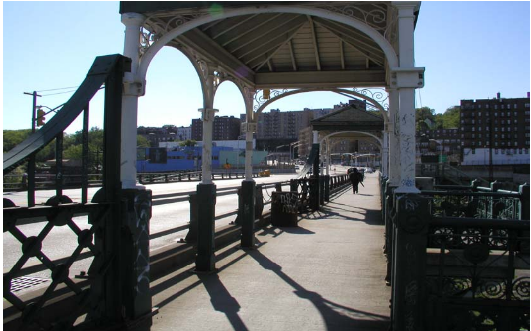
University Heights Bridge near Fordham Landing
