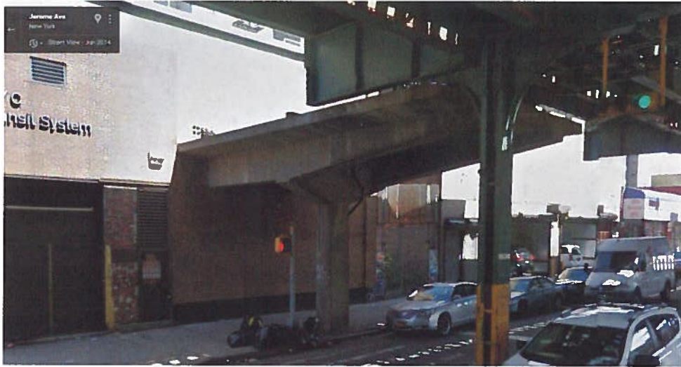
Figure 11: Jerome Avenue at West 176th Street
