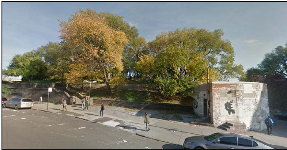
3) Croton Aqueduct System (resource below-grade, portion of Aqueduct Walk public park visible in photo)
