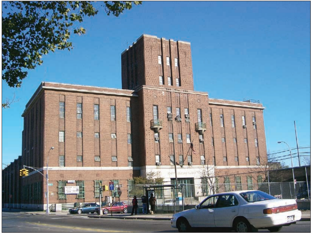
104th Field Artillery Armory (23). View southwest 22
