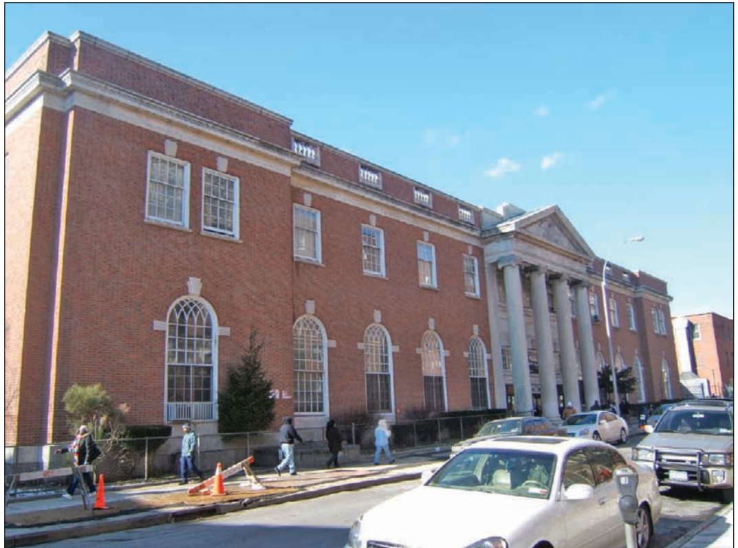
Jamaica Post Office (17). View northwest 15
