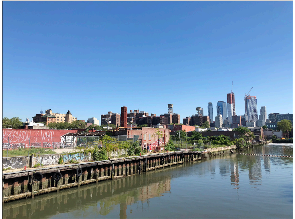
Buildings in the S/NR-eligible Gowanus Canal Historic District along the west side of the Canal Aa
