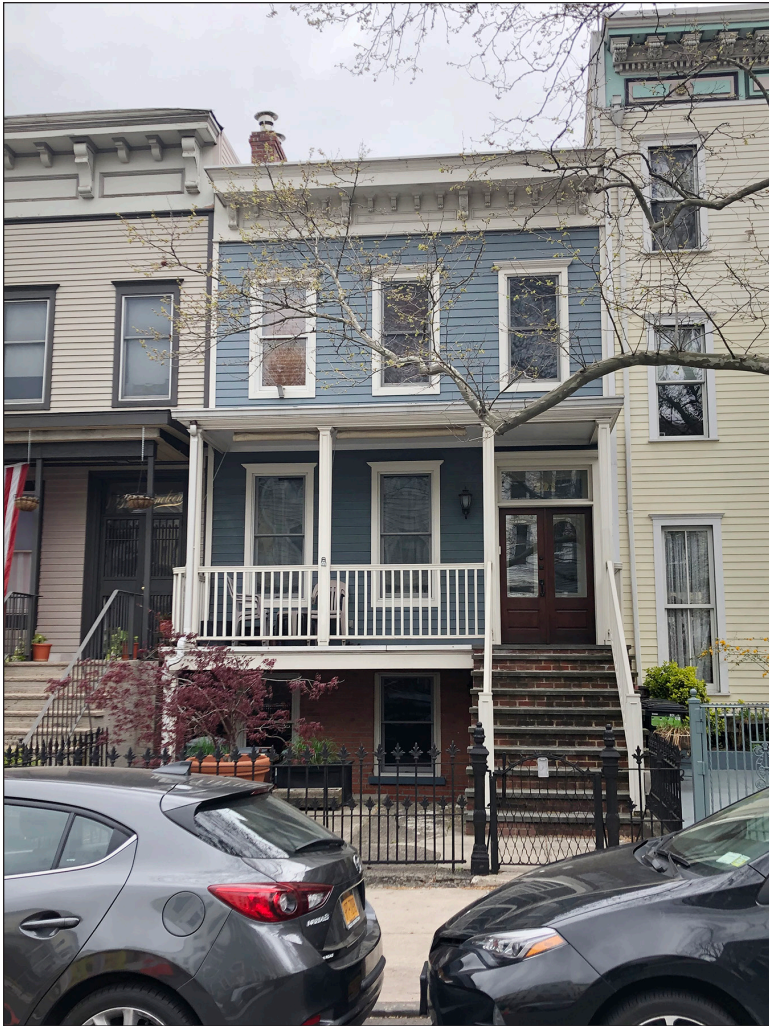
Wood-frame house at 221 11th Street [S/NR-eligible] 28e
