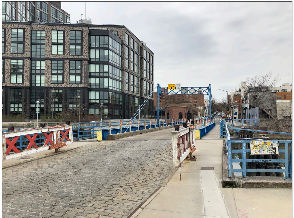
The Carroll Street bridge & Operator's House [S/NR-eligible, NYCL] 6
