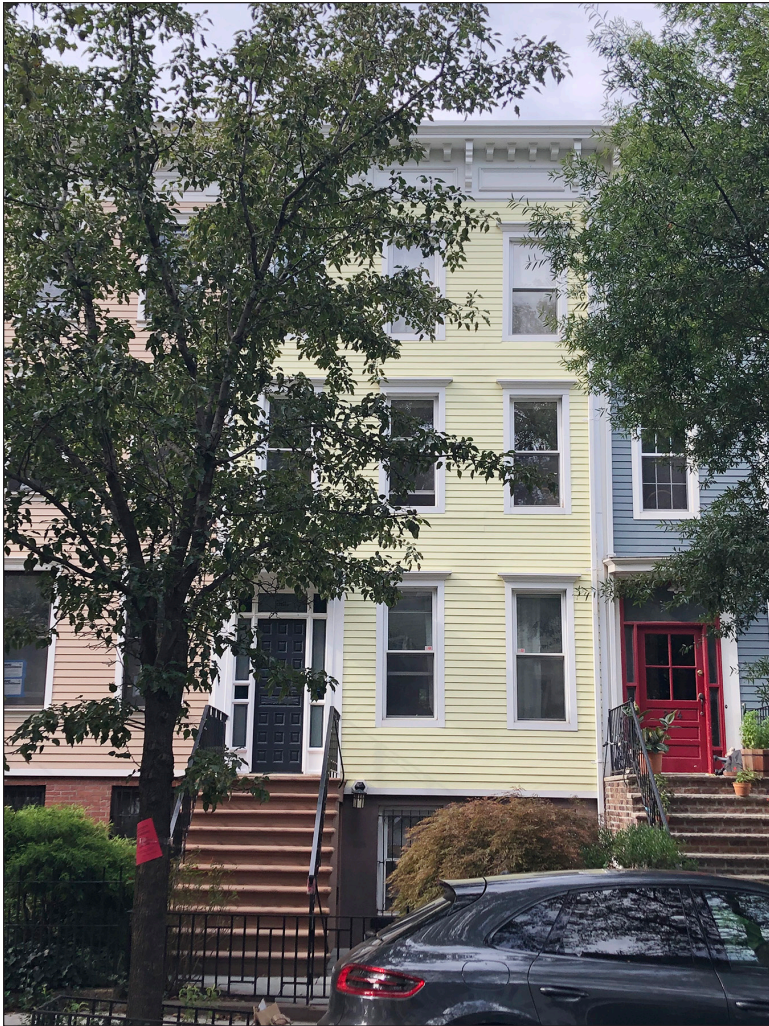
Wood-frame house at 226 11th Street [S/NR-eligible] 28g
