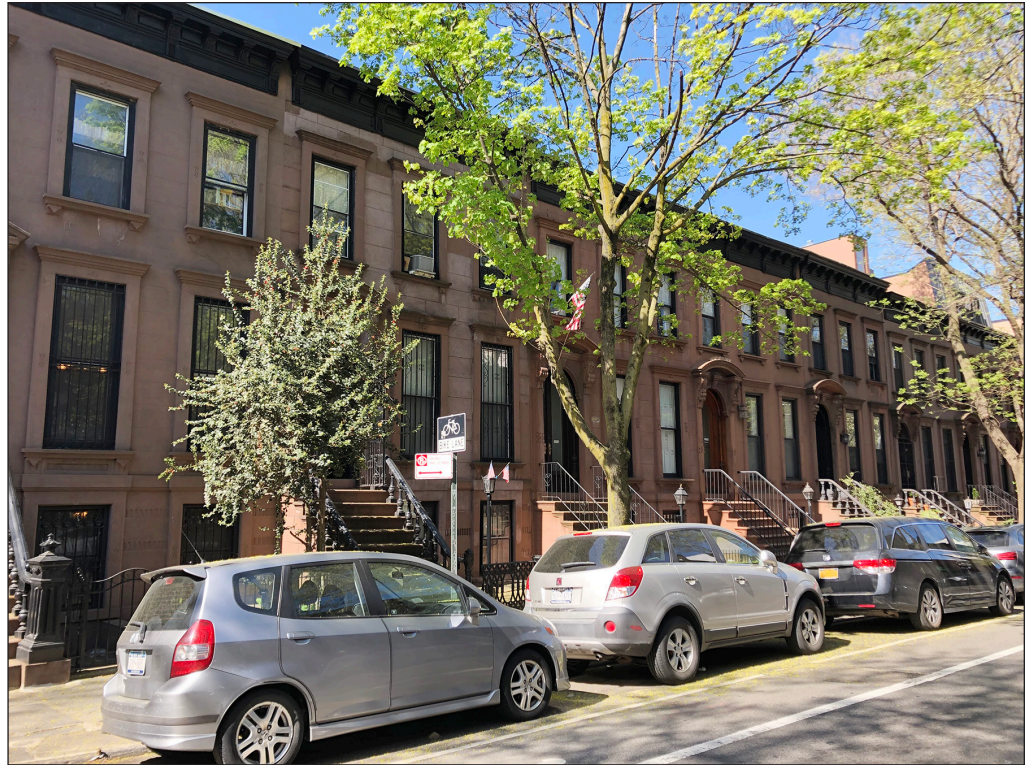
Five of the twenty row houses at 376-414 Bergen Street [S/NR-eligible] 17
