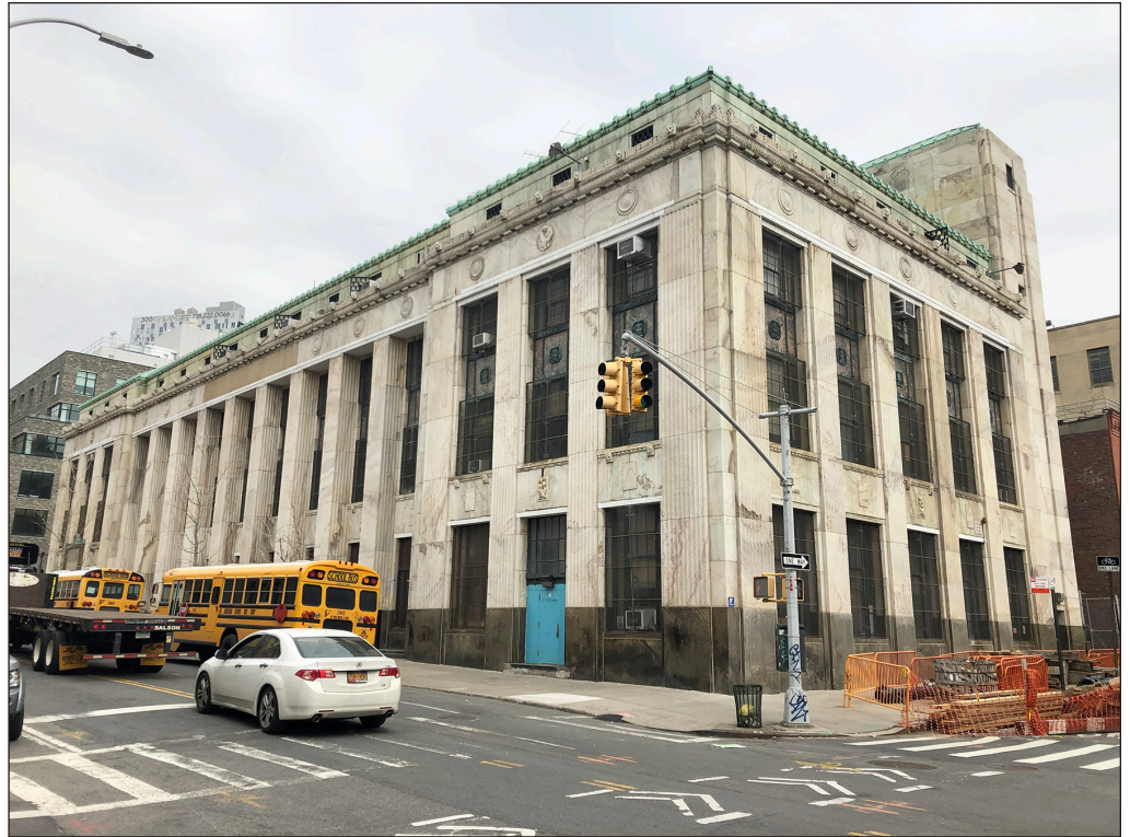
Former Brooklyn Printing Plant of the New York Times [S/NR-eligible, NYCL-eligible] 19 at 59-75 3rd Avenue
