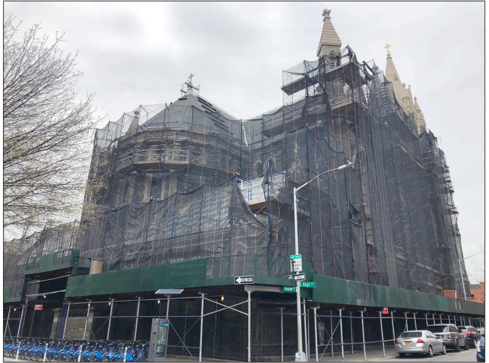
St. Agnes Church [S/NR-eligible, NYCL-eligible] at 267-285 Hoyt Street 21a
