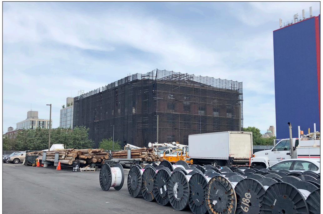
Former BRT Power House [S/NR-eligible, NYCL] at 153 2nd Street 12
