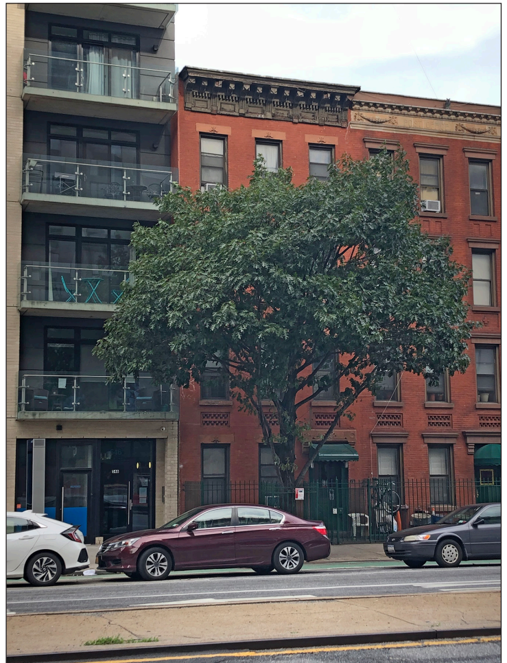
Row house at 544 4th Avenue [S/NR-eligible] 2
