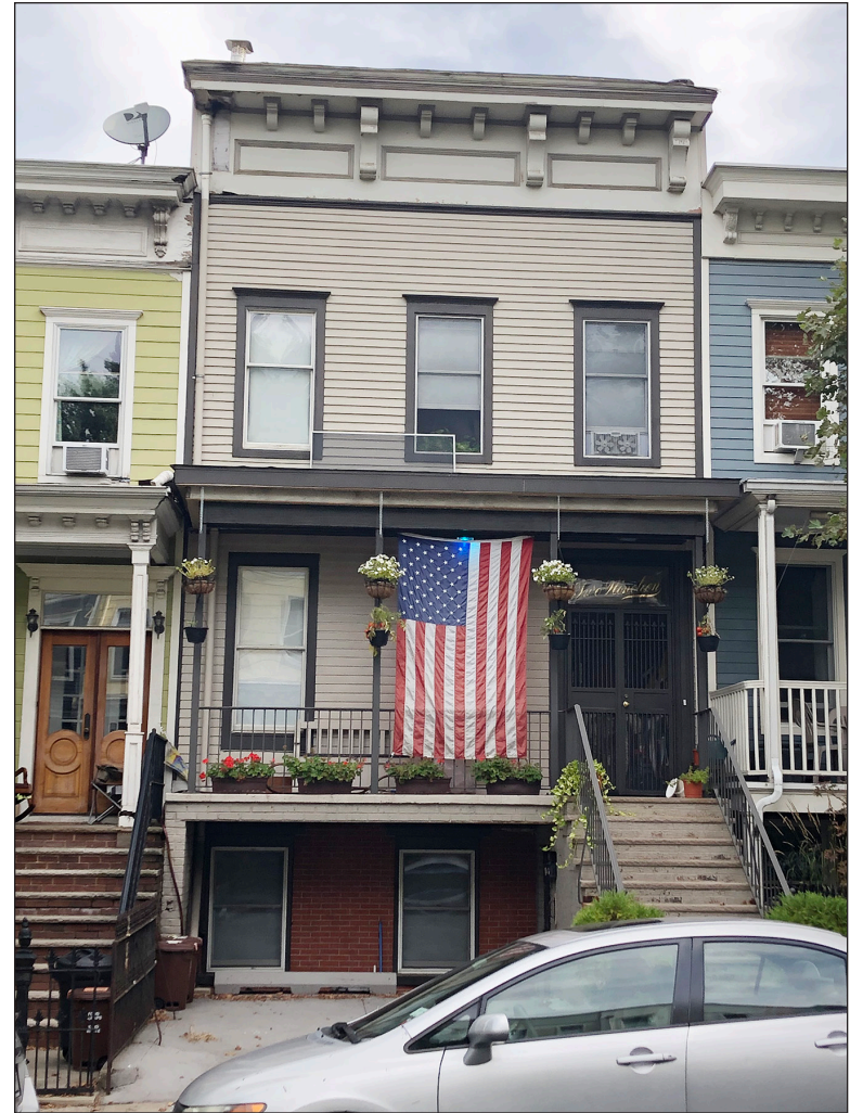
Wood-frame house at 219 11th Street [S/NR-eligible] 28d
