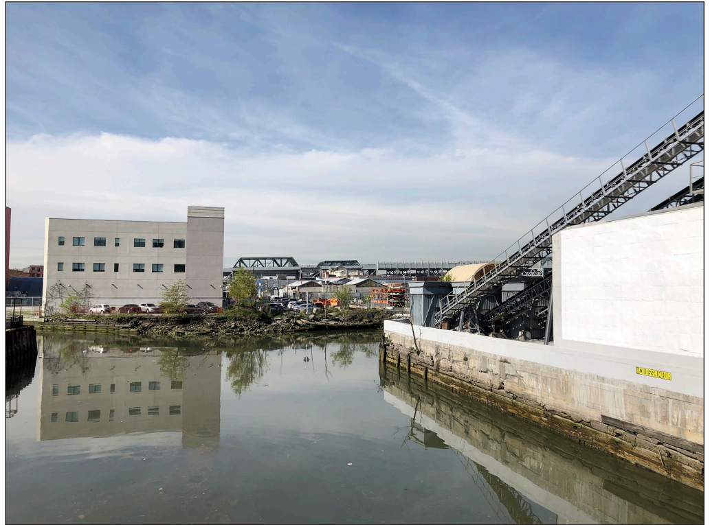
View south from the 3rd Street bridge of the Canal and buildings in the Gowanus Canal Historic District Ac
