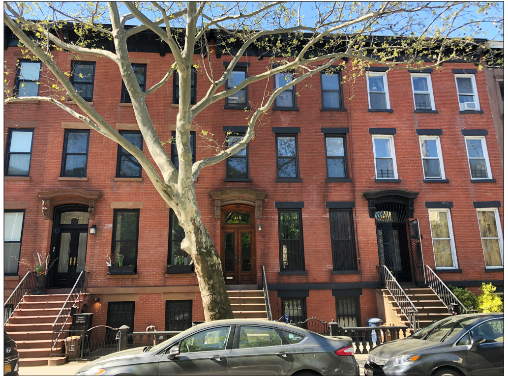
Three of the ten Italianate row houses at 398-418 Dean Street [S/NR-eligible] 15
