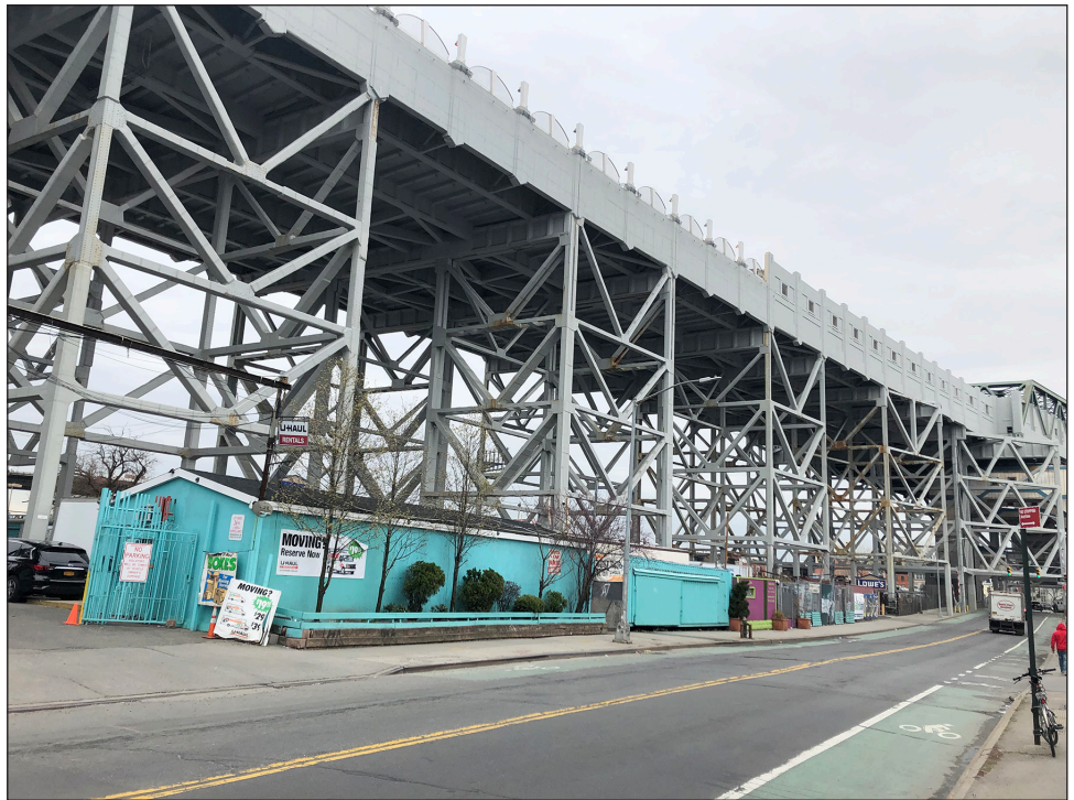
The IND Subway Viaduct [S/NR-eligible] between Smith Street and 3rd Avenue, north of 10th Street 27
