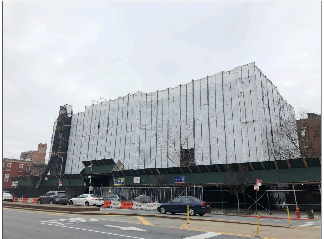
Public School 124 [S/NR-eligible] at 515 4th Avenue 11
