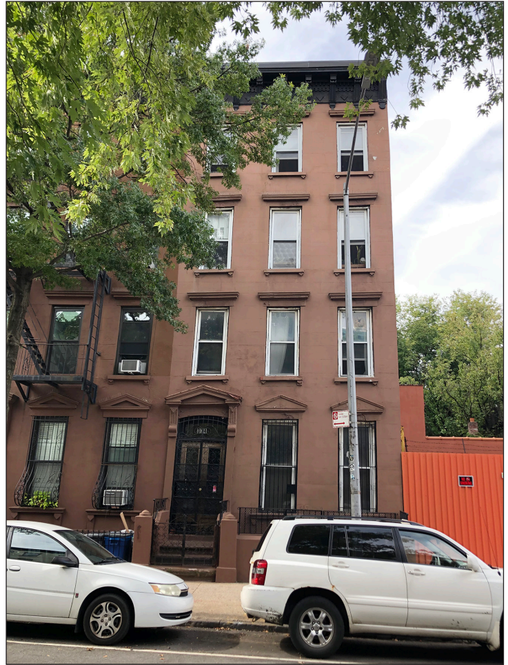
Row house at 374 Bergen Street [S/NR-eligible] 5
