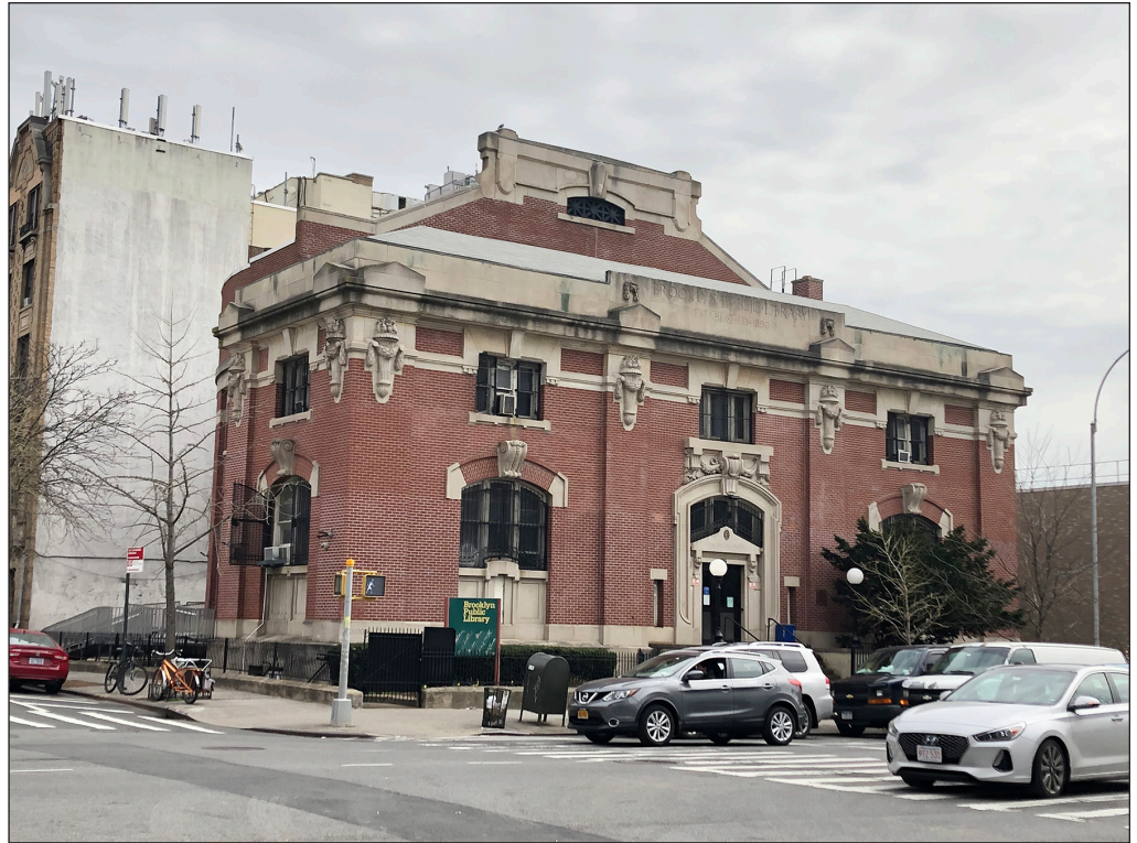
The Brooklyn Public Library, Pacific Branch [S/NR-eligible, NYCL-eligible] 3 at 25 4th Avenue
