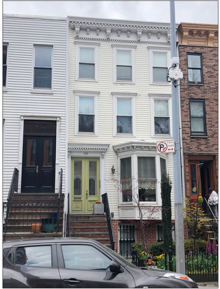
Wood-frame house at 232 11th Street [S/NR-eligible] 28i
