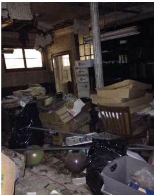
Photo 29: Storage room in the eastern portion/rear of the basement.
