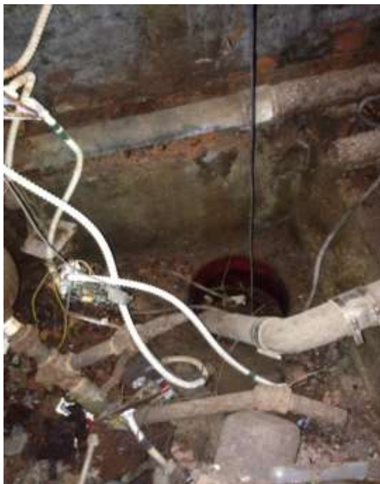
Photo 25: Sump located in the boiler room.
