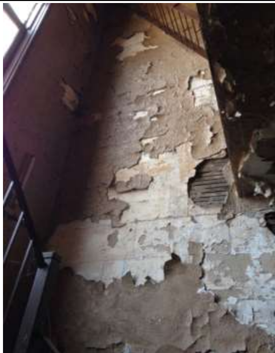
Photo 22: Typical conditions of the interior painted surfaces in the synagogue.
