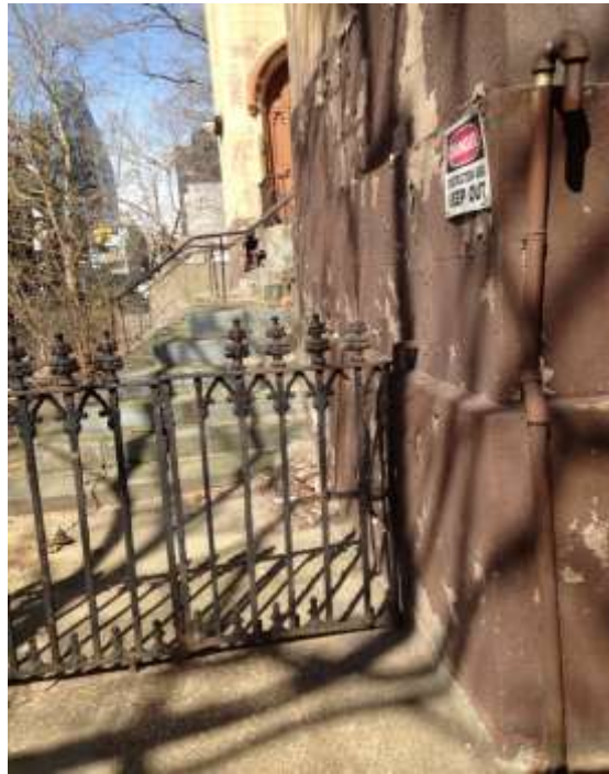
Photo 3: Fuel oil fill port and vent pipe in the sidewalk in front of the southwestern corner of the synagogue on the subject property on Lot 37.
