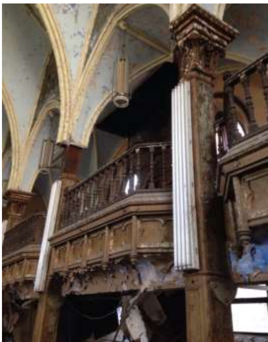
Photo 30: Lighting ballasts on the first floor of the synagogue.
