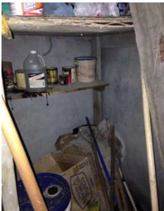
Photo 28: Chemical storage in the basement outside of the boiler room.
