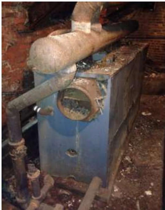
Photo 24: Boiler room located in the basement in the southwestern corner of the synagogue.
