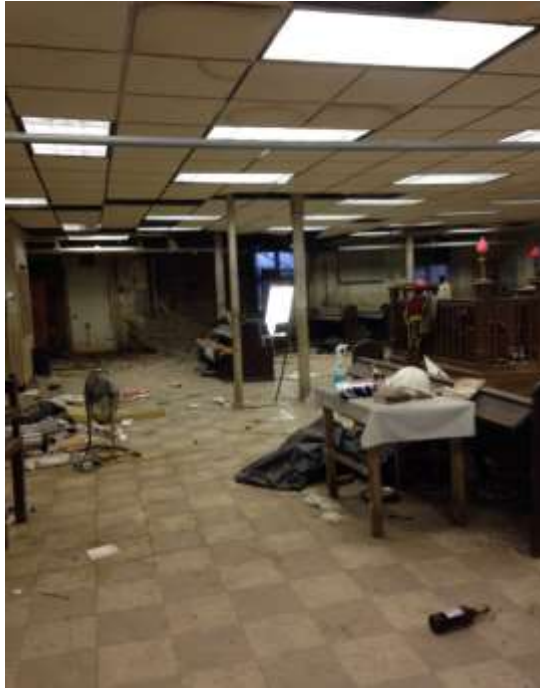
Photo 23: Interior of the basement of the synagogue located on the subject property at Lot 37.
