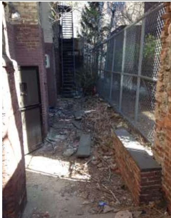
Photo 4: Alley on the southern portion of Lot 37 and access to the basement level of the synagogue, facing east.
