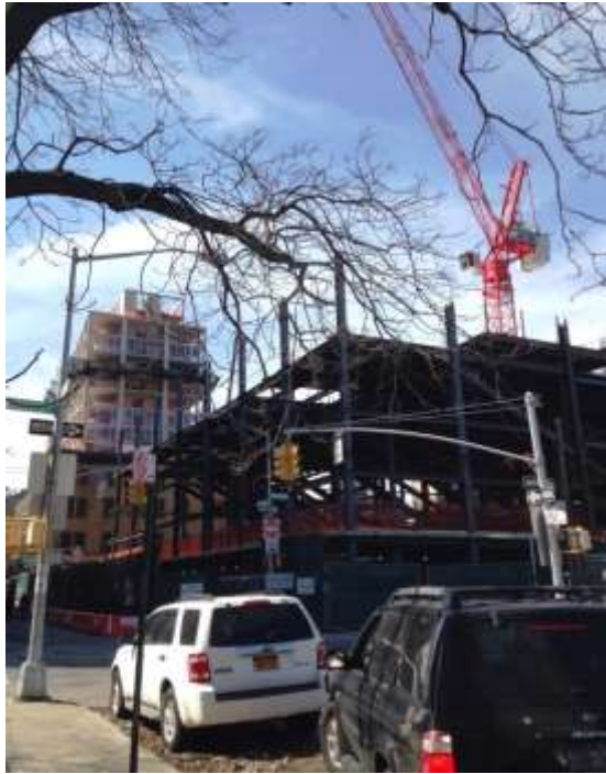
Photo 15: Active redevelopment site across the intersection of Norfolk Street and Broome Street from the subject property, facing northwest.
