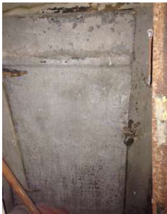
Photo 26: Locked door immediately to the south of the boiler room. Suspected location of the fuel oil storage tank.
