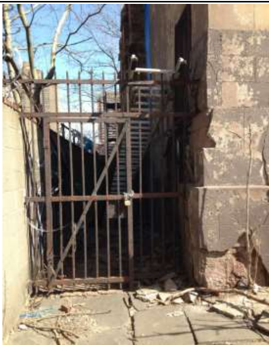
Photo 5: Alley on the northern portion of Lot 37, facing east. Inaccessible during site reconnaissance.
