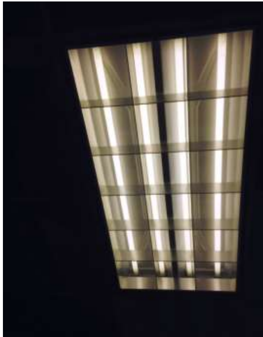
Photo 31: Lighting ballasts in the basement of the synagogue.
