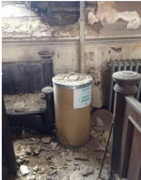
Interior of the first floor of the synagogue located on the subject property at Lot 37. A Photo 21: container of sweeping compound, a petroleum-based product, is located in the northeast corner.
