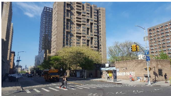
View north along Essex St from its intersection with Grand St. Seward Park Extension NYCHA is a 23-story development within the project area.
