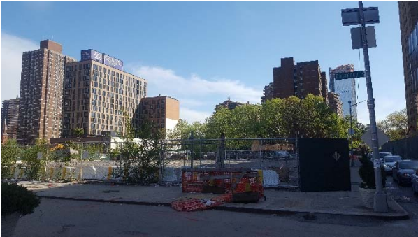
View south from Delancey St near its intersection with Norfolk St towards the Affected Area.
