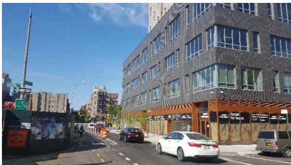
View north from Clinton St/ Broome St southwest corner. Essex Crossing Site 6 is shown on right.
