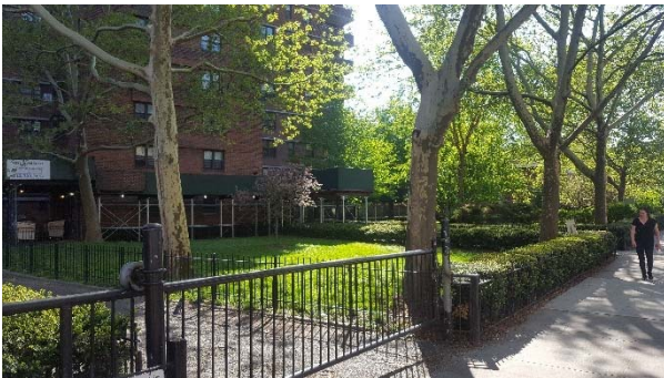
View southwest from Grand St near its intersection with Suffolk St. The setback creates a "Tower in the Park" setting.
