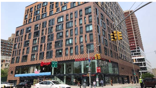
Essex Crossing Site 5, as seen from southeast corner of Grand St/ Clinton St. The building is completed.
