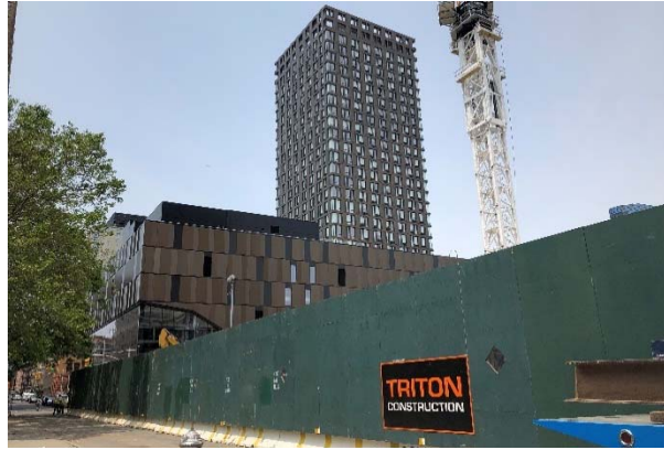
View northwest from southwest corner of Broome St/Suffolk St. Essex Crossing Site 2 is shown center. Essex Crossing Site 3, under construction, is shown right.
