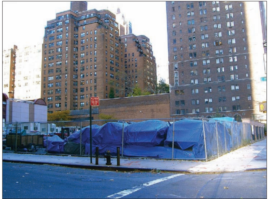
685 First Avenue development parcel. View northwest from East 39th Street at First Avenue 3
