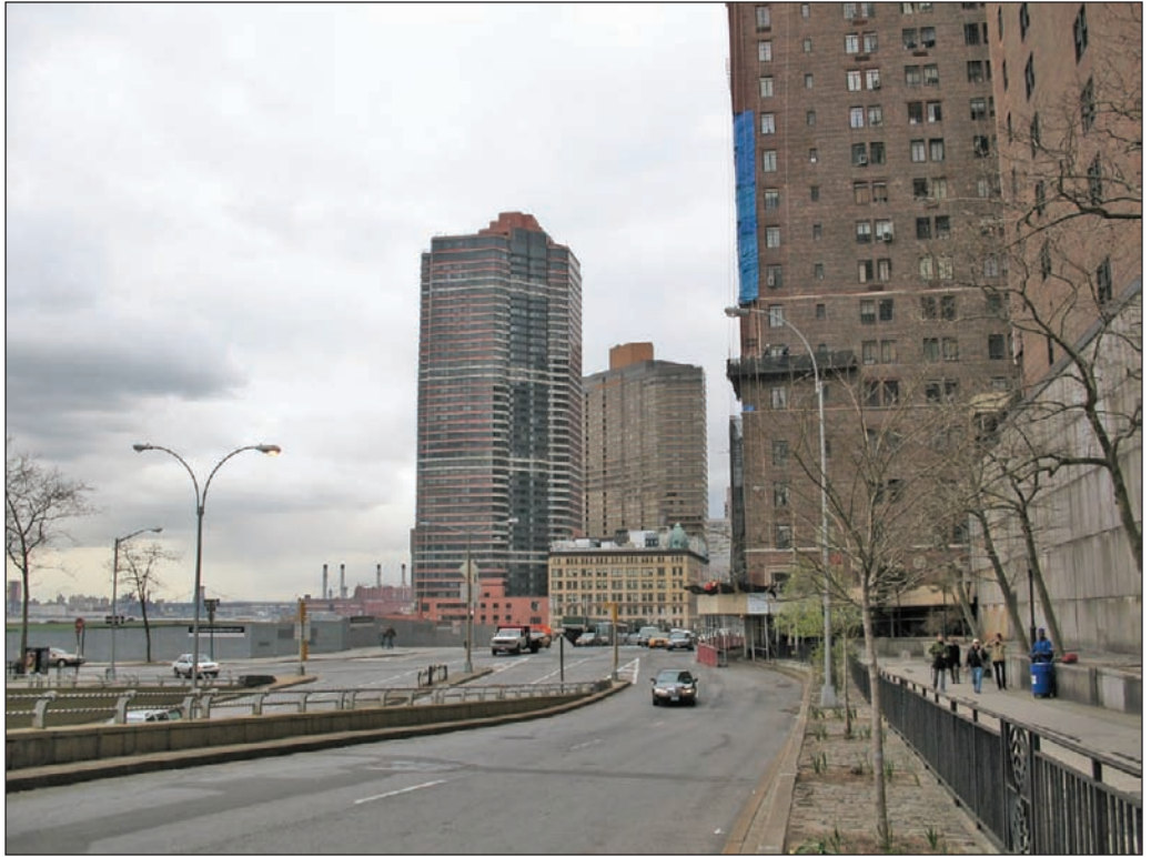
Waterside and 708 First Avenue development parcels. View south on First Avenue from East 42nd Street 5
