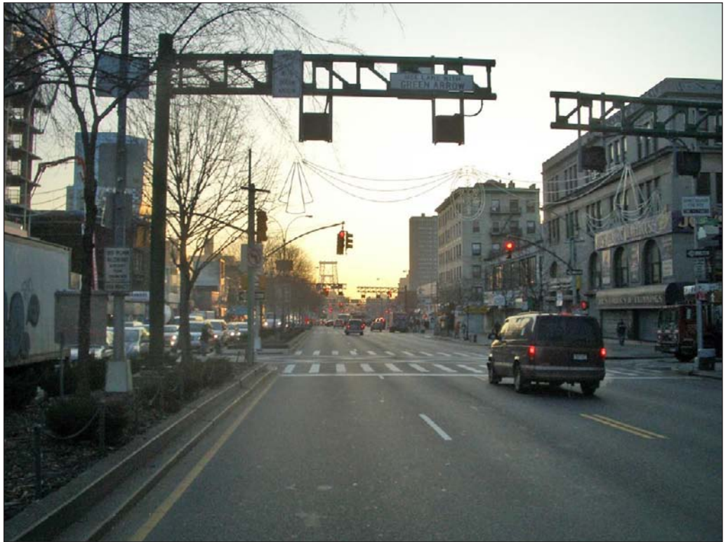
View east of Delancey Street at Allen Street 45 (Williamsburg Bridge in background)
