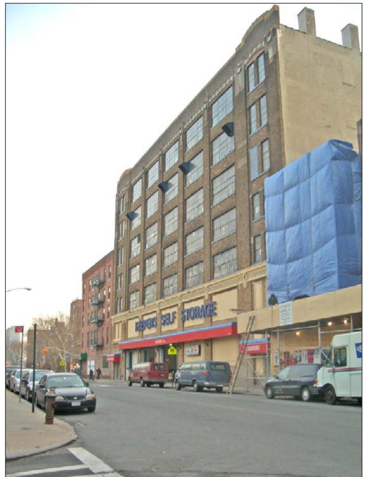
View of the south side of East 10th Street east of Szold Place 16
