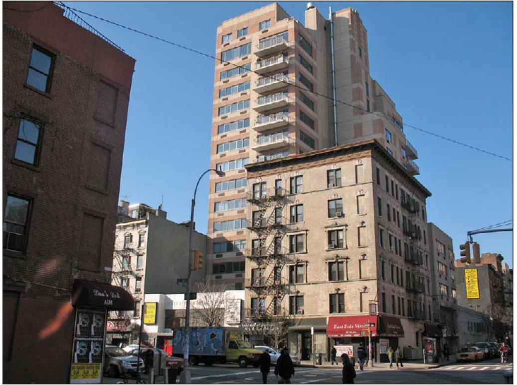
View of the west side of First Avenue between East 9th and East 10th Streets 7
