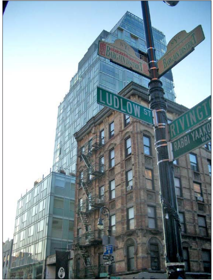
View of the Hotel on Rivington from Rivington and Ludlow Streets 33
