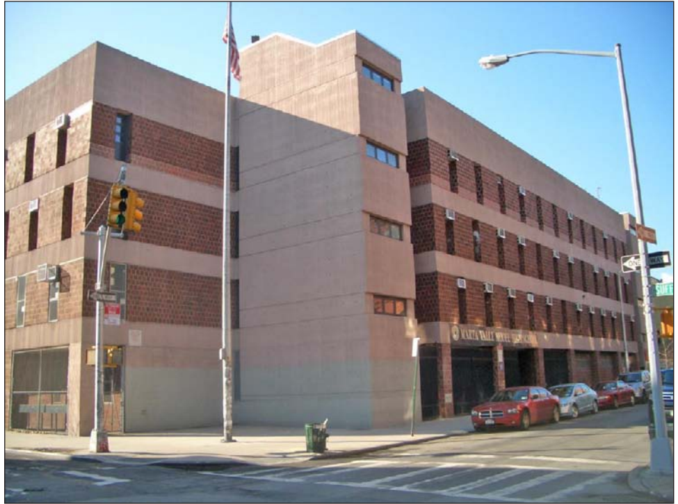
The Lower East Side Preparatory School and the Marta Valle School at 145 Stanton Street 39
