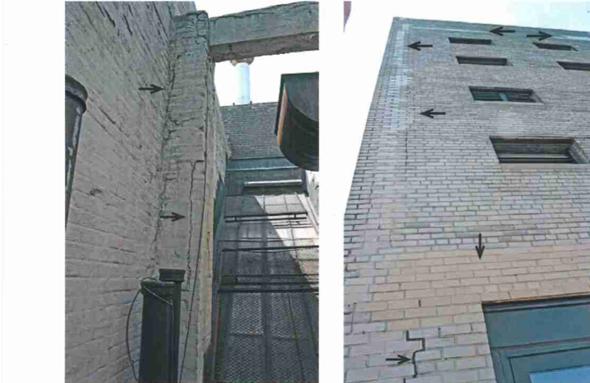
At top of building there is visible evidence of vertical cracks in the brick barrier wall construction where moisture has penetrated into the masonry and damaged the steel behind. The image on the right shows mis-matched brick repairs and on-going vertical cracks.
