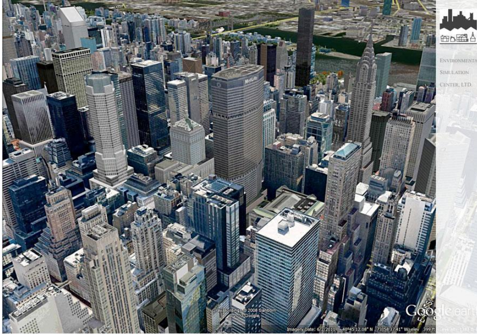
View of East Midtown from the Southwest – Existing Conditions
