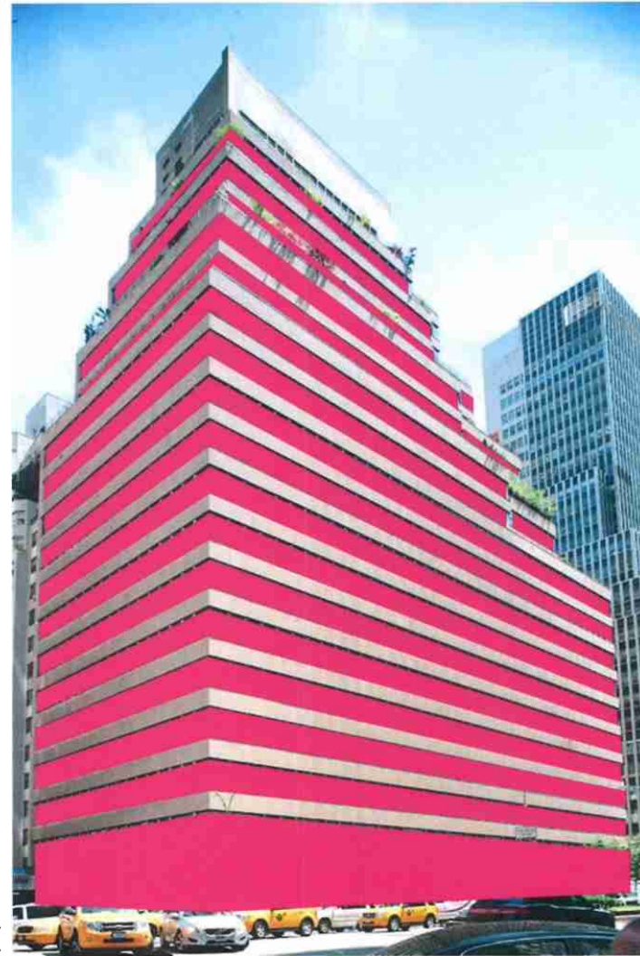
2013: alterations to the original exterior building fabric that affect the building's physical integrity
