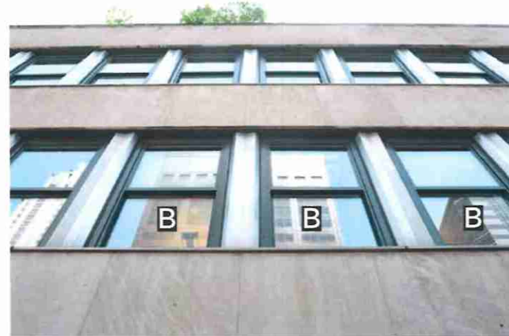
Top shows original steel window with narrow frame profile: ● Bottom shows modern wide aluminum window frame profiles. The original alternating A-B-A pattern is now B-B-B.
