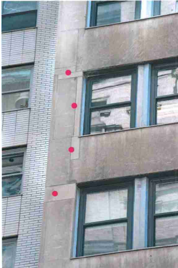
● Patchwork limestone repairs
