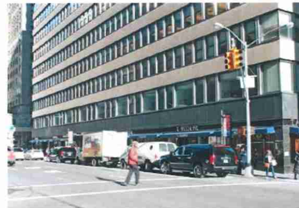
New dark stone base replaces original limestone panels
