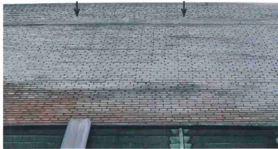
Bulges in the brick masonry of the cooling tower are suggestive of deterioration that will need expensive repair.
