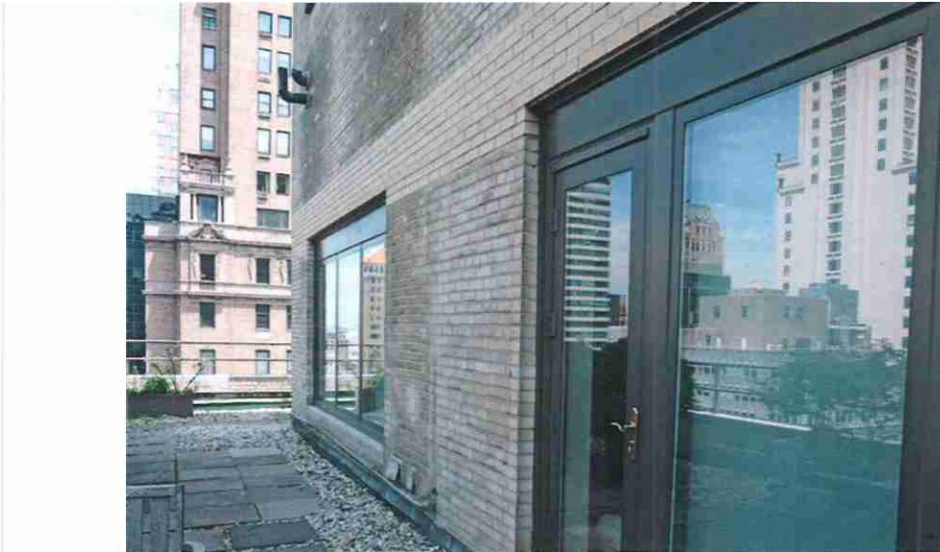
Modern aluminum windows and door system at upper level.
