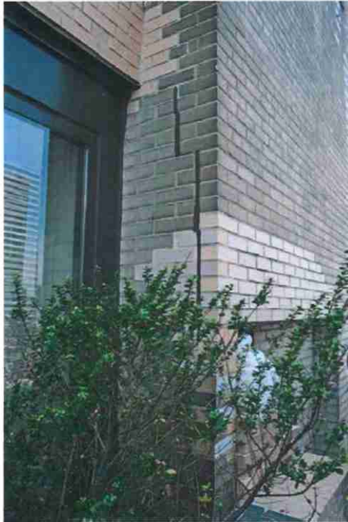
Mis-matched brick repairs and vertical cracks in masonry at corner
