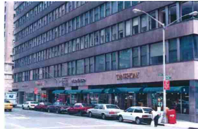
Original limestone panels and stainless steel storefront base
