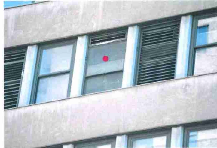
Top shows original steel window with narrow frame profile: ● Bottom shows modern wide aluminum window frame profiles. The original alternating A-B-A pattern is now B-B-B.
