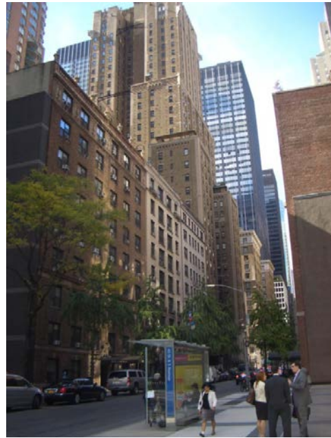
10: View of the built context along East 49 th Street, looking west from Third Avenue
