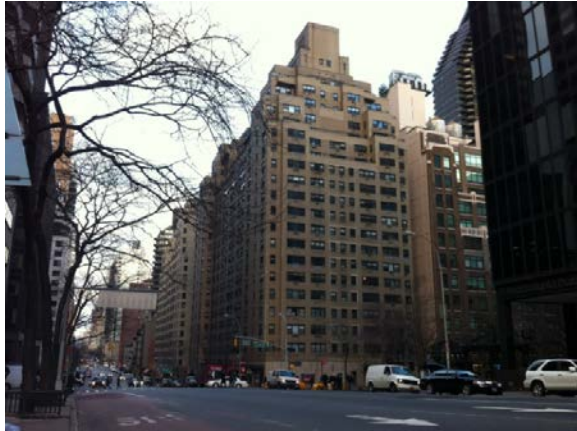
5. View of the built context along Second Avenue, looking north from East 46 th Street
