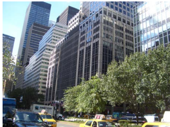
8. View of the built context along Park Avenue, looking south from East 52 nd Street
