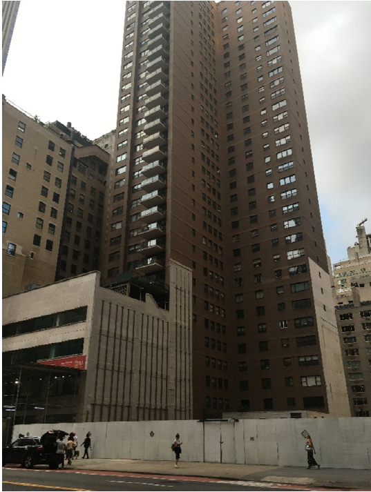
Photo 1 West 57th Street between Fifth and Sixth Avenues Looking Northwest
