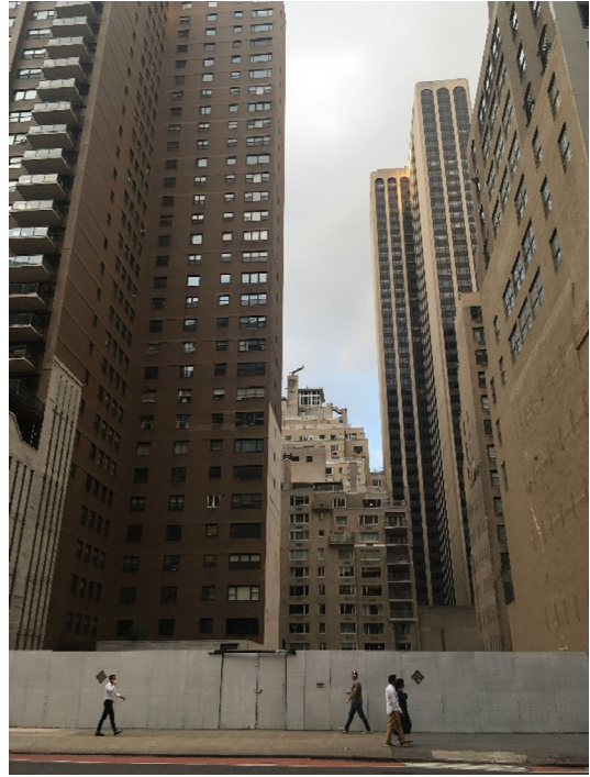
Photo 2 West 57th Street between Fifth and Sixth Avenues Looking North
