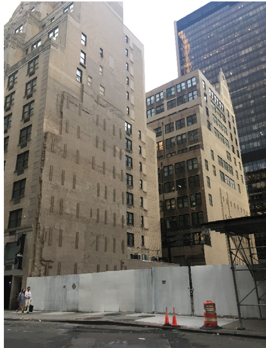
Photo 4 West 58th Street between Fifth and Sixth Avenues Looking Southeast
