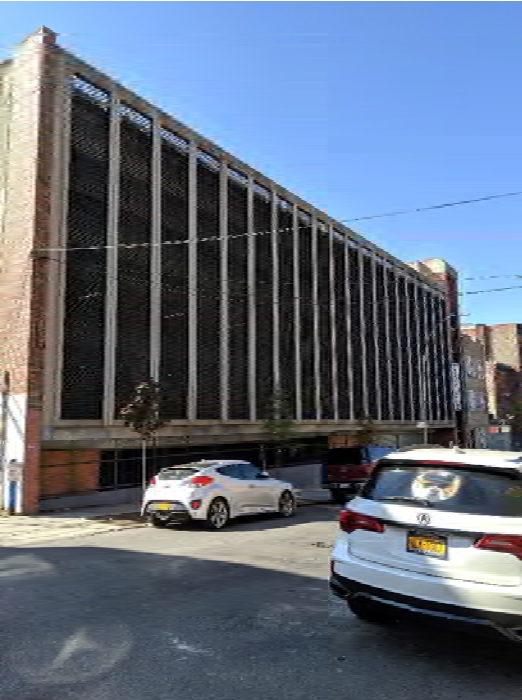
Photo 6-7 Municipal Parking, view looking southwest on East 150th St
