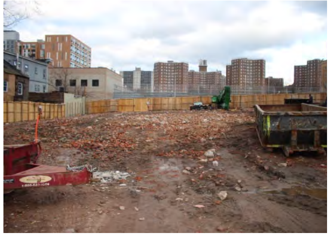
Photo 2. View of Development Site 1 looking north from East 150th Street
