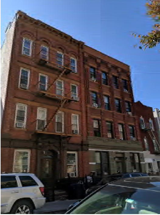
Photo 6-5 View looking southwest on East 151st St, near Courtlandt Ave
