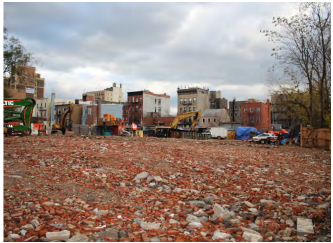
Photo 4. View of project area looking south on East 151st Street
