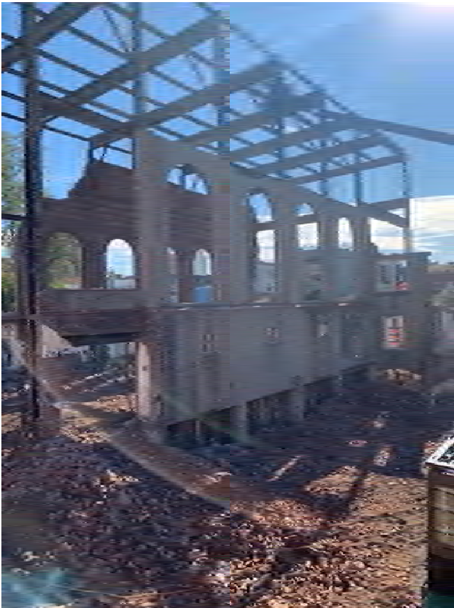
Photo captured 11/5/20 prior to complete demolition
