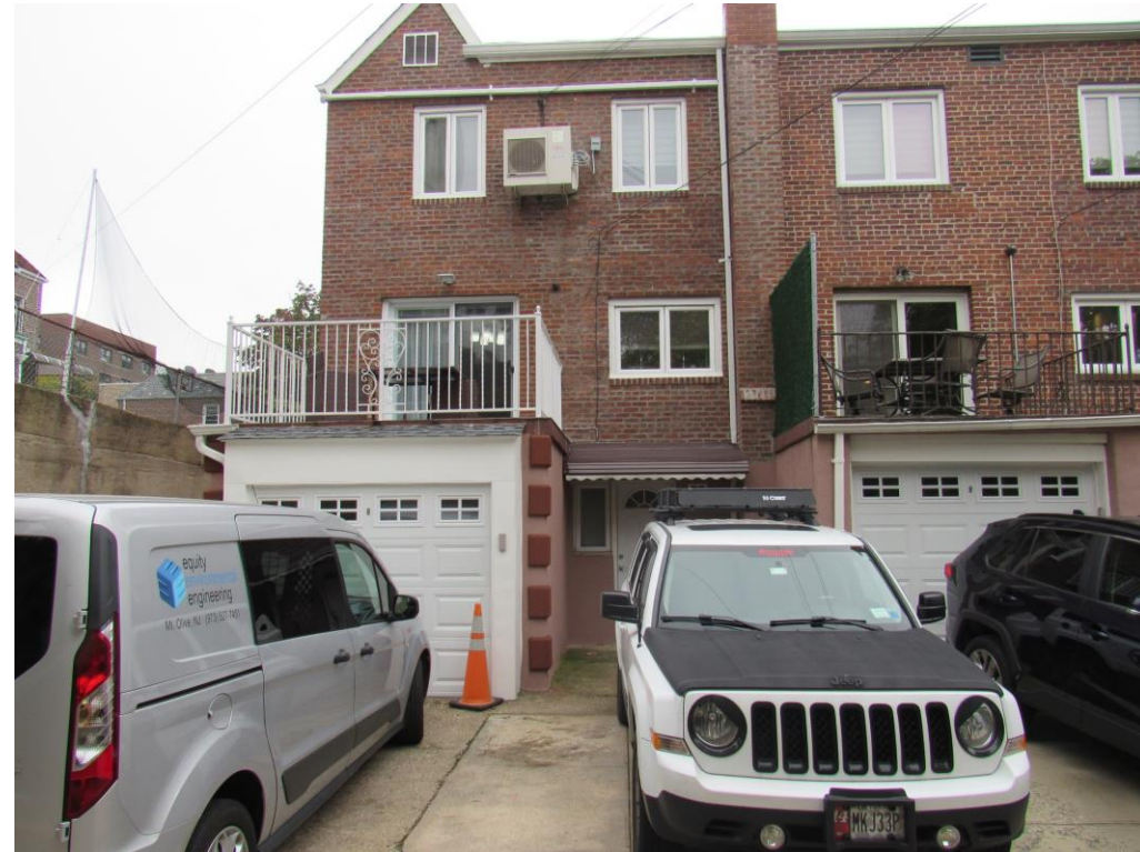
05 VIEW OF THE REAR OF THE SUBJECT PROPERTY
