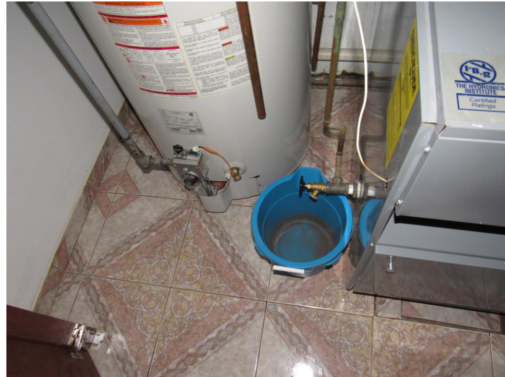
09 VIEW OF THE BOILER AND HOT WATER HEATER CLOSET IN 66-45 WETHEROLE STREET
