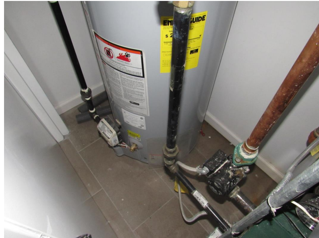
13 VIEW OF THE BOILER AND HOT WATER HEATER CLOSET IN 66-47 WETHEROLE STREET
