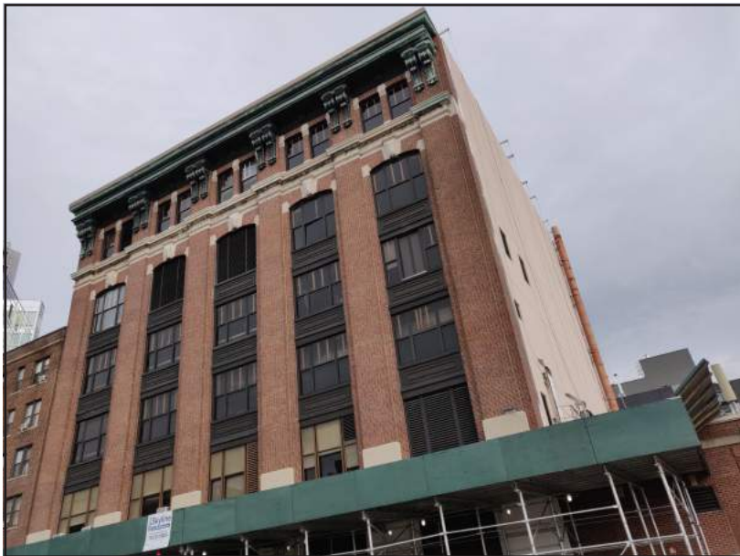
Resource #4: Telephone Building at 547-555 Clinton Avenue.
