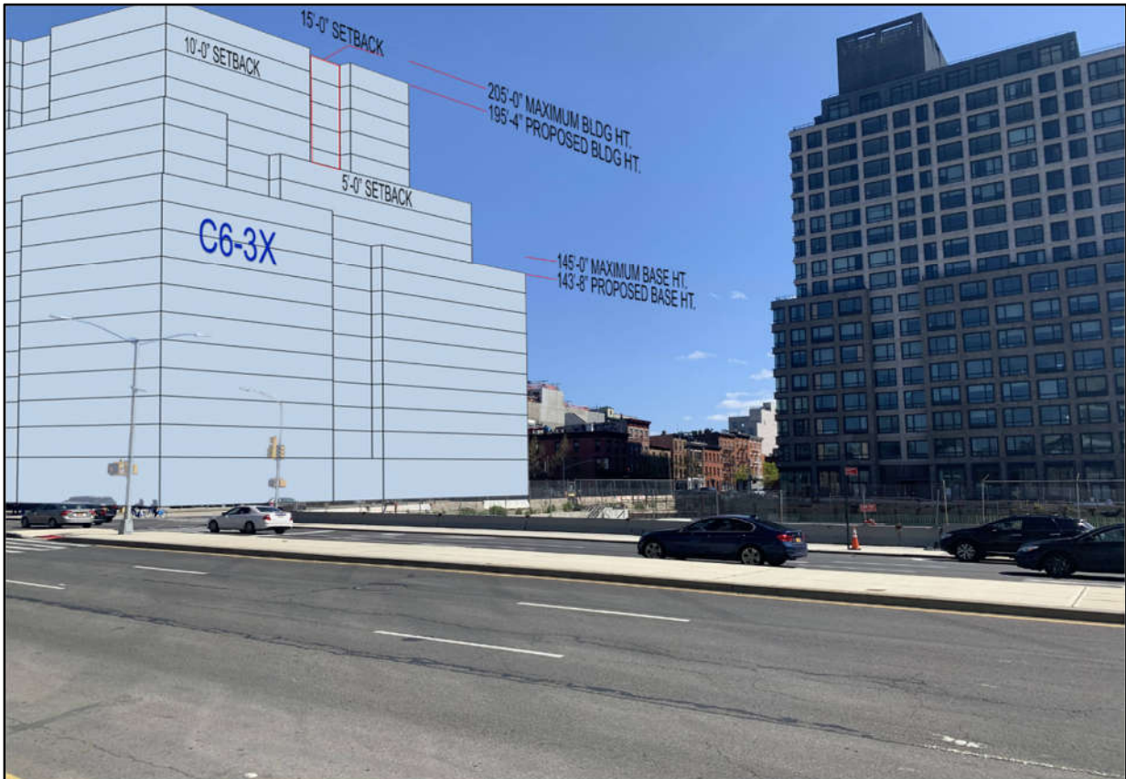
With-Action condition on the Development Site looking south east along Atlantic Avenue.
