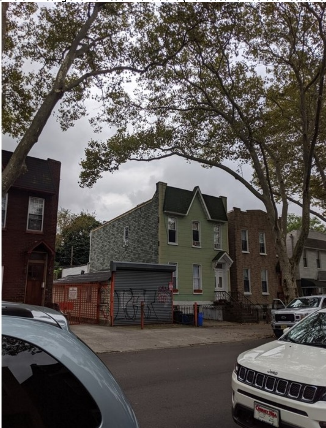
Figure 2.3-3: Existing and No-Action Conditions (View east from across Decatur Street)
