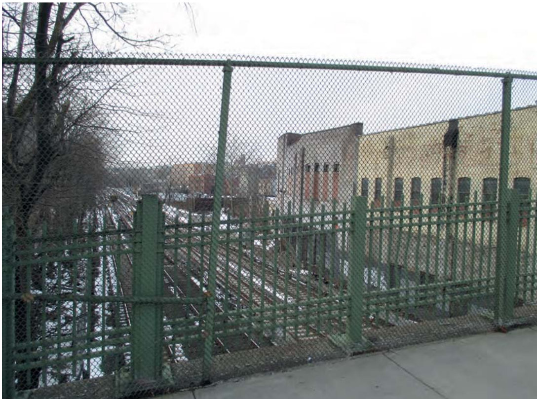
6. Looking west towards rear of project site from Bedford Park Boulevard railroad overpass
