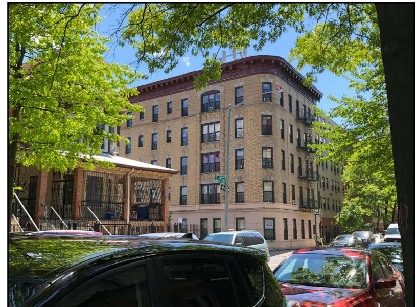
10) Looking south from Decatur Avenue towards East 199th Street.
