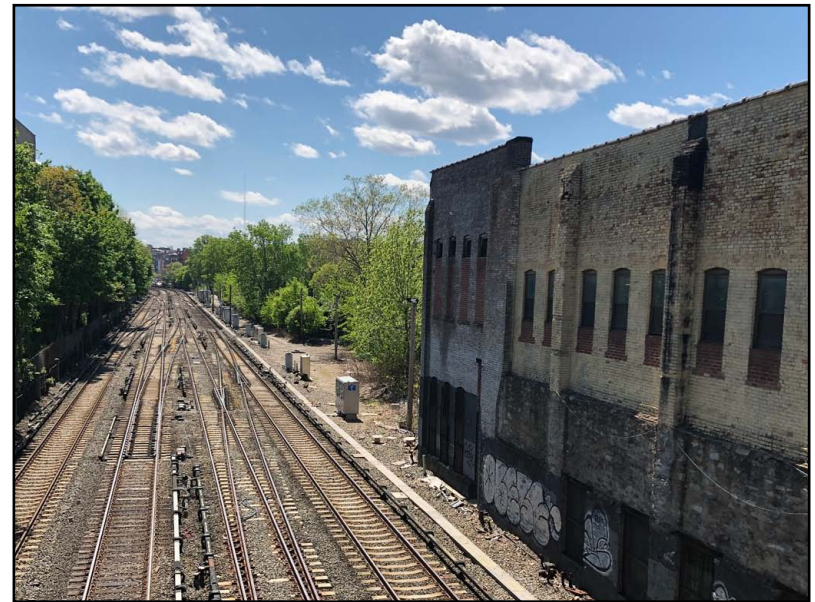
4) Looking west from Bedford Park Boulevard toward the southeastern facade of the Project Site and the MTA Metro North Harlem Line tracks.
