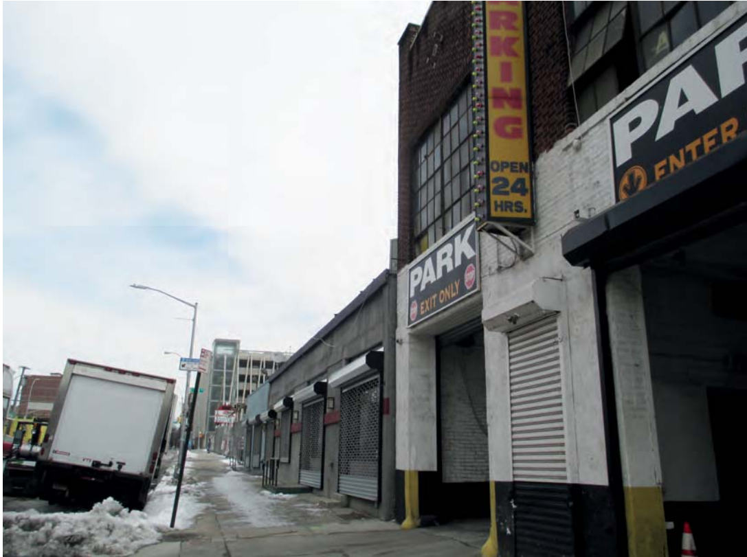
7. Looking north along Webster Avenue towards project site
