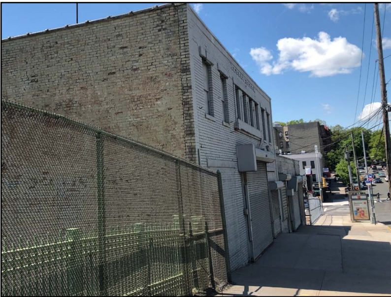
3) Looking northwest towards the Project Site from Bedford Park Boulevard.
