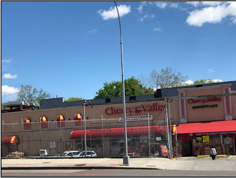
1) Looking southeast from Webster Avenue towards Lots 122 and 128 on the Project Site.
