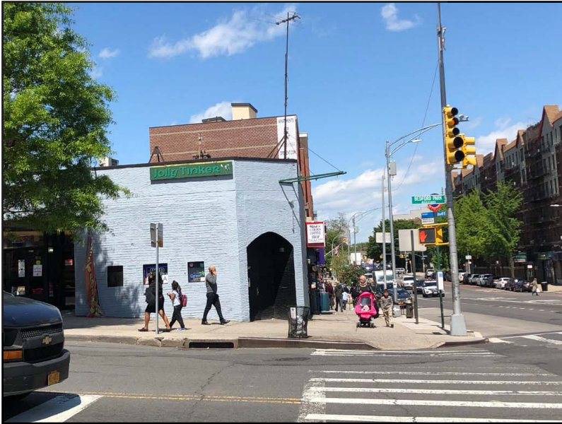
9) Looking northeast from the intersection of Webster Avenue and Bedford Park Boulevard.
