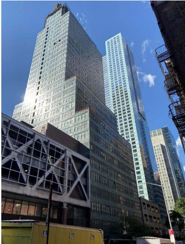
Photograph C-5: View of the McGraw-Hill Building from Eighth Avenue
