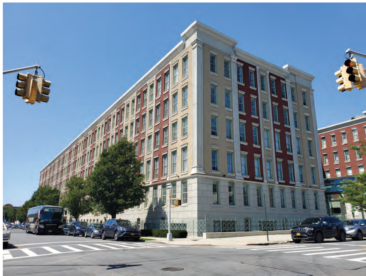
15. View of the Project Area facing west from the intersection of Ditmars Boulevard and 46th Street.
