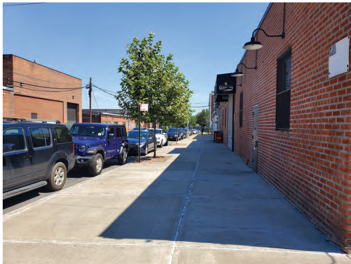
45. View of the sidewalk along the southeast side of 45th Street facing northeast from 23rd Avenue (Project Area at right).
