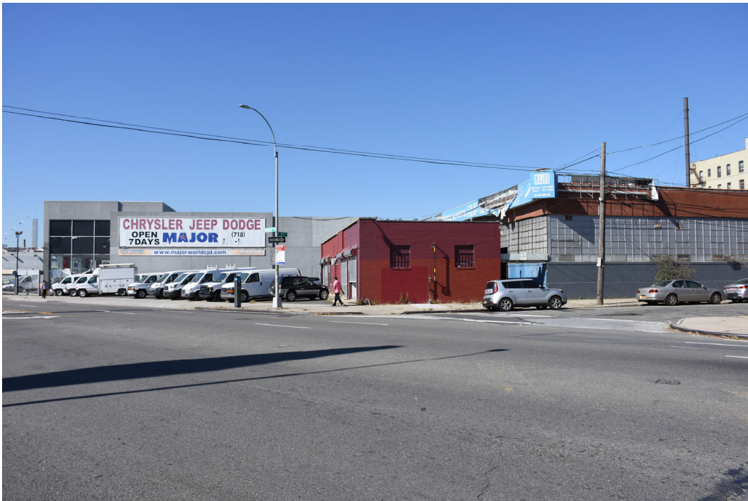
Photo 2: View of project site from Northern Boulevard, between 45 th and 46 th Streets looking northwest.
