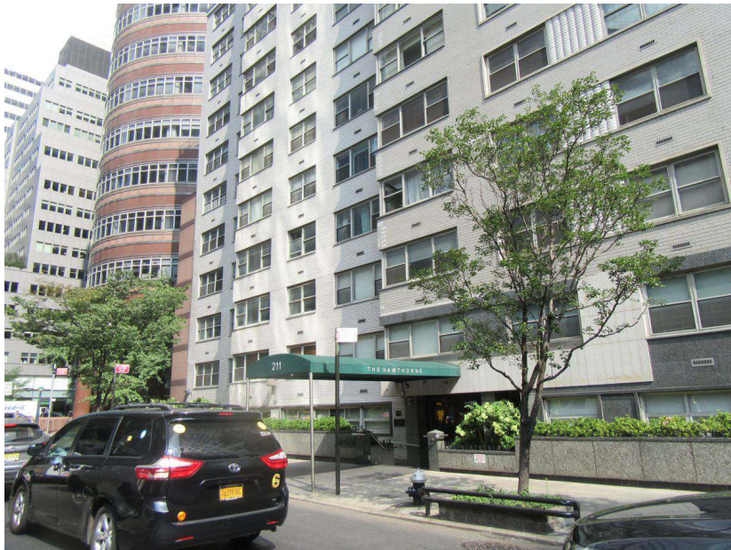
6. View of the side of East 53rd Street facing northwest between Second Avenue and Third Avenue.
