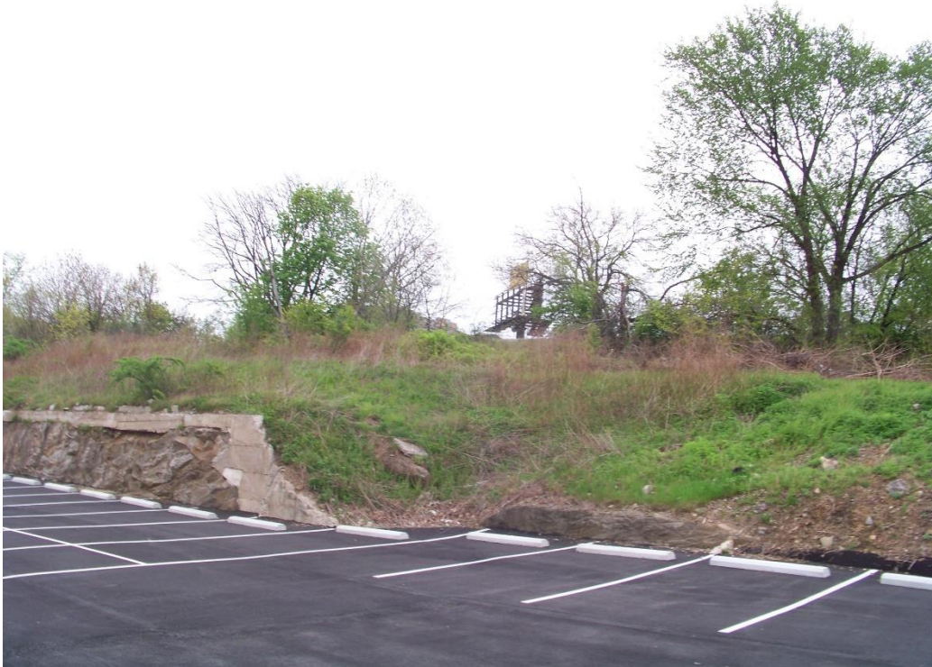
Wooded buffer between Applicant's Property and the Bronx River Parkway
