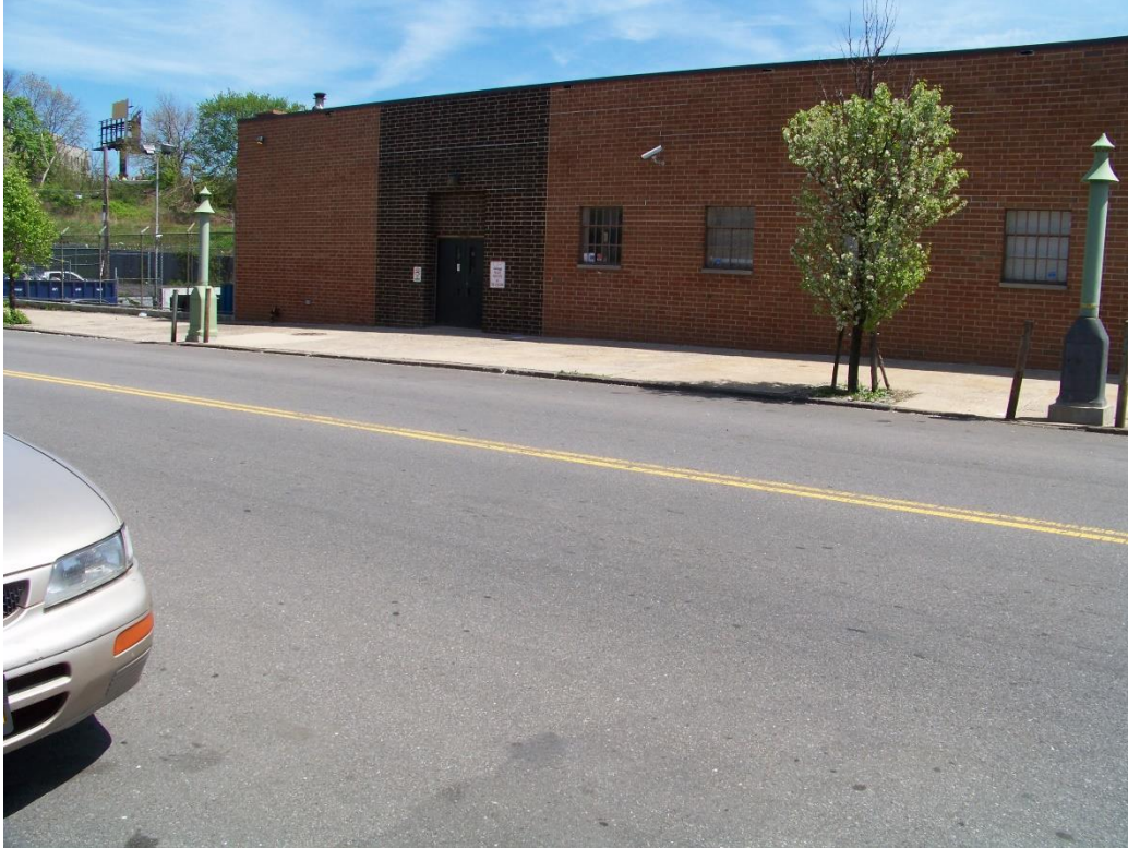
Warehouse development south of affected area
