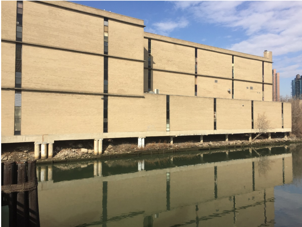
Photo 5: Views of building's eastern façade adjacent to Dutch Kills
