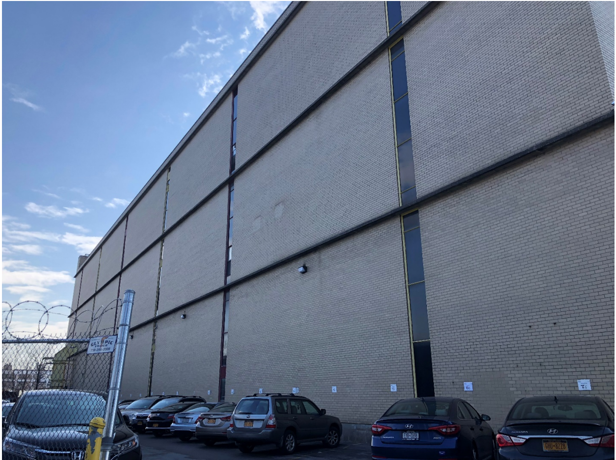
Photo 10: View of building's northern façade from 27 th St
