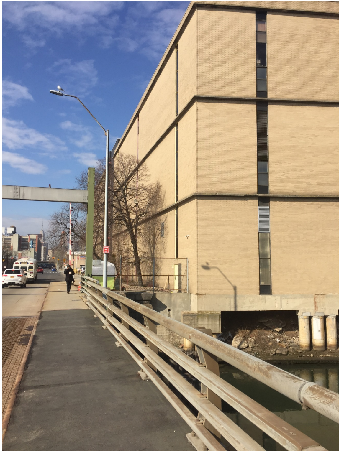
Photo 6: View of building facing west on 49 th /Hunters Point Ave
