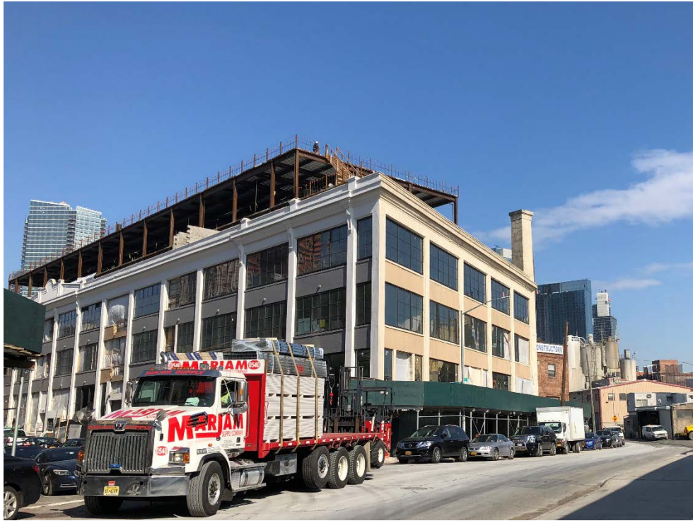
View of a 3-story former manufacturing (office conversion) building on 27 th Street undergoing a vertical enlargement (Block 97, Lot 4)
