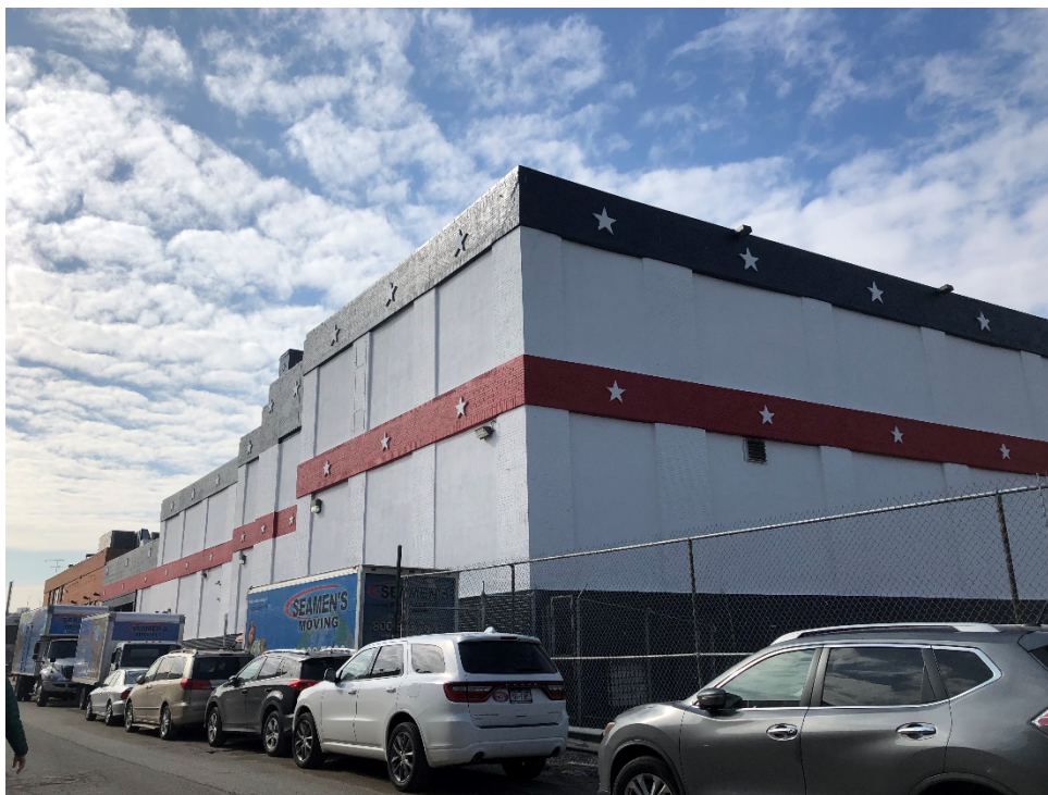
View of a taller, 3-story brick warehouse in the study area, which is located along 29 th street (Block 115 Lot 249)
