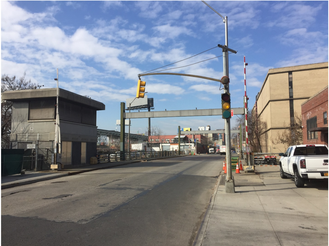
Photo 4: View of bridge and project site on 49 th /Hunters Point Ave
