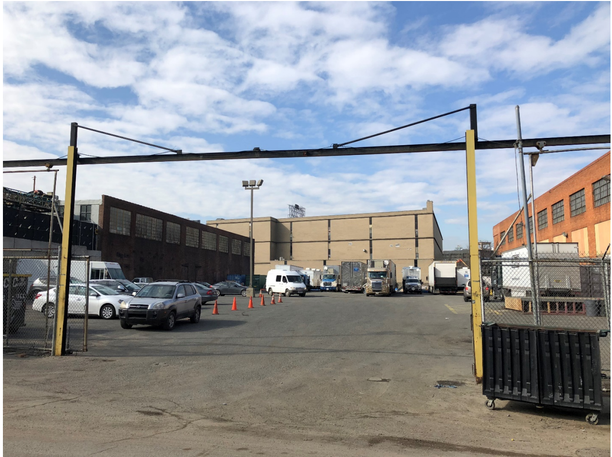
Photo 2: View of the building's eastern façade from 30 th Street
