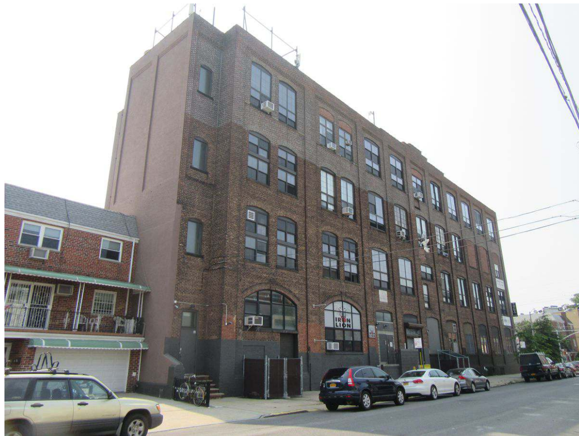
4. View of Projected Development Site 1 facing south from 38th Street.
