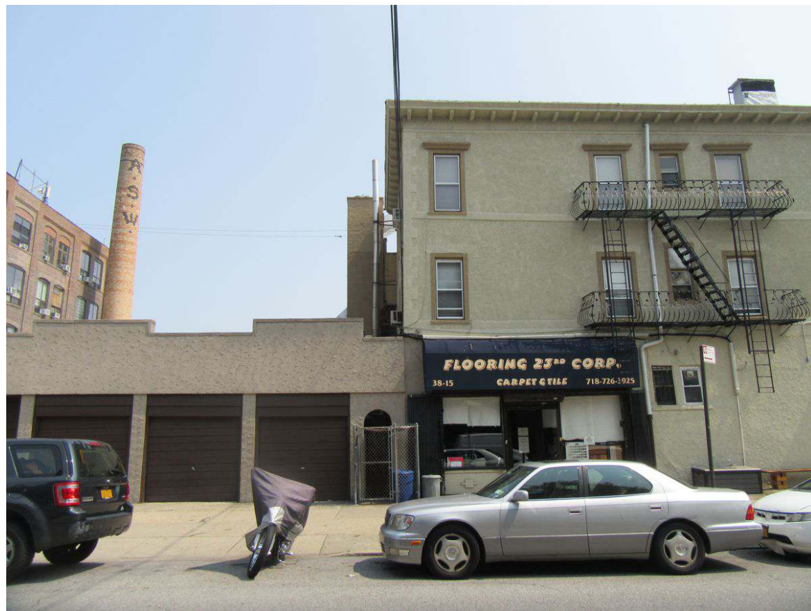
19. View of Other Site 1 facing northeast from 23rd Street.
