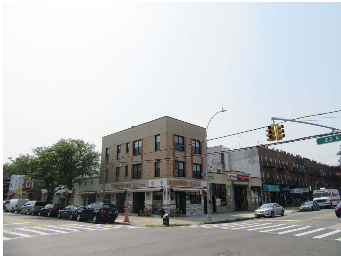
33. View of the intersection of 23rd Avenue and Steinway Street facing south from Other Site 1.
