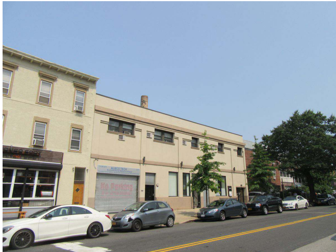
22. View of Projected Development Site 2 facing north from Steinway Street.
