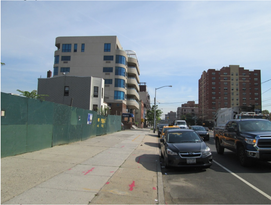
Looking north on 21 st Street from 31 st Avenue toward the development site.
