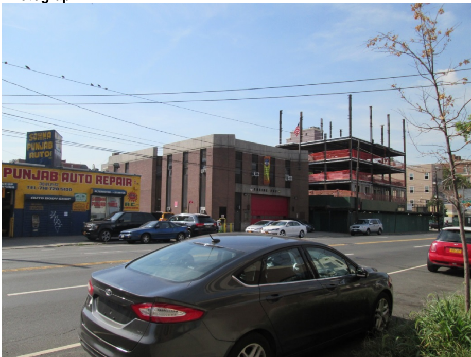
Midblock on 21 st Street looking east, just south of 30 th Drive.
