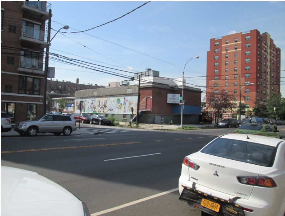
Looking south on 21 st Street toward the existing Variety Boys and Girls Club and 11-story residential building.
