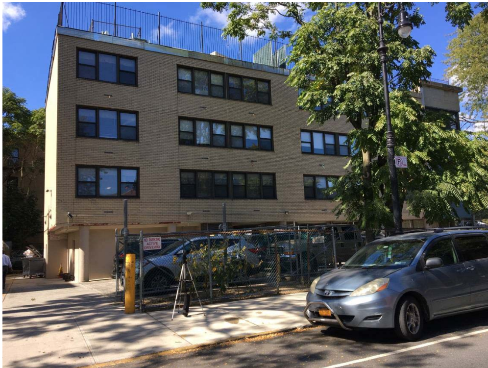
Meter Setup at Location 2
