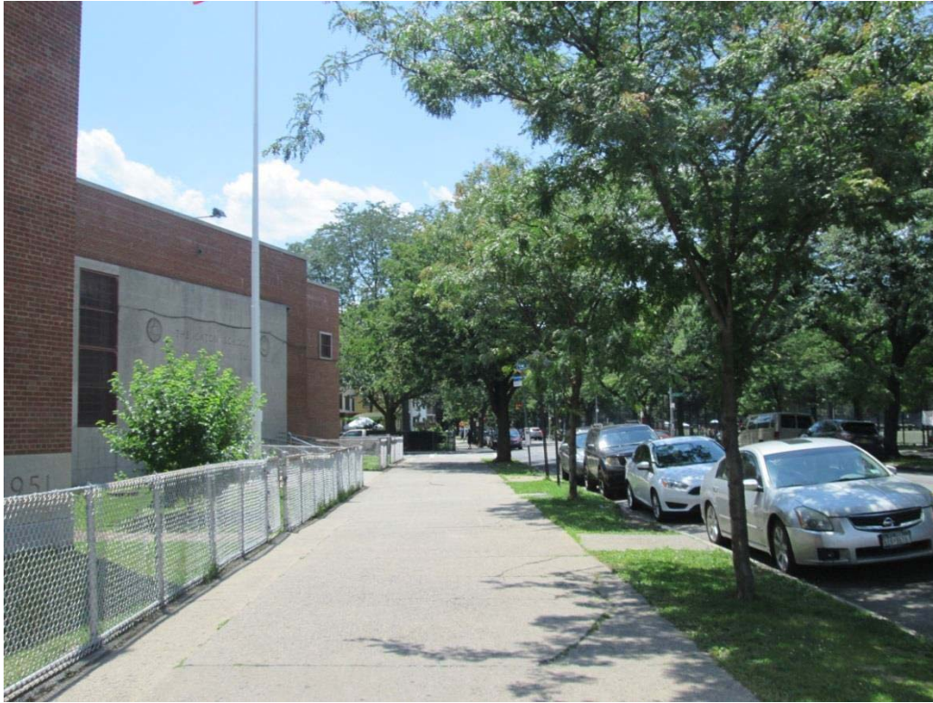
Photo 5: View of The Caton School (PS 249) from the midblock point between Rugby Road and Marlborough Road on Caton Avenue facing southwest.
