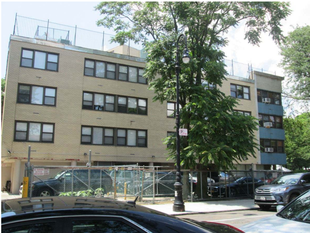
Photo 10 Close up view of Nursing Home from Rugby Road looking west
