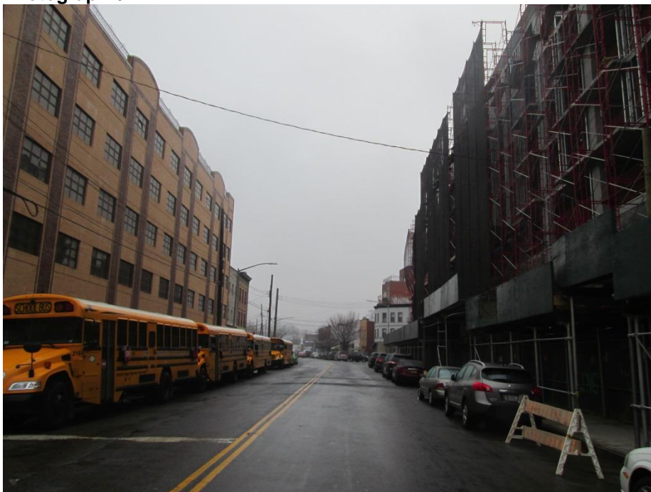
Looking north on New Utrecht Avenue towards 40 th Street with new development on the right hand side of the street
