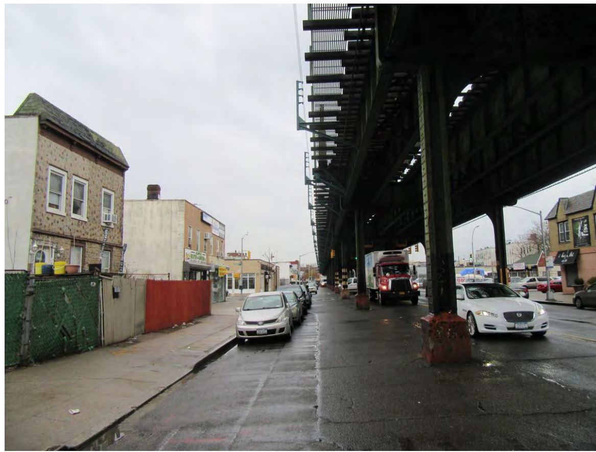
4. View of McDonald Avenue facing south (Site at left).
