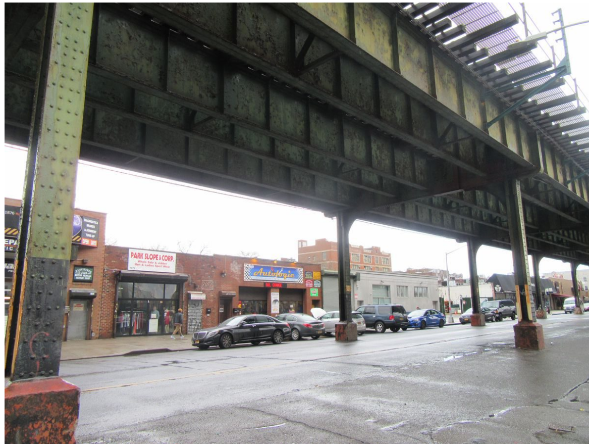
3. View of the side of McDonald Avenue facing northwest from the Site.
