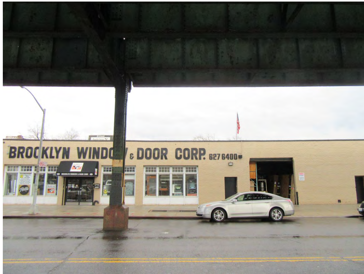
24. View of the side of McDonald Avenue facing east between Quentin Road and Woodside Avenue.
