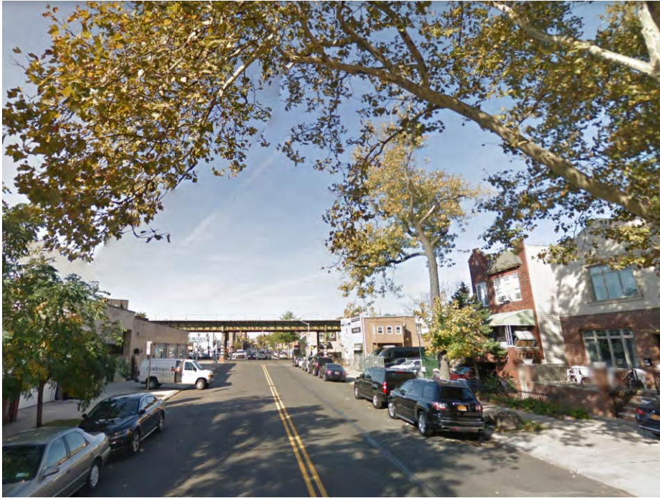
Quentin Road facing west (Site at right)
