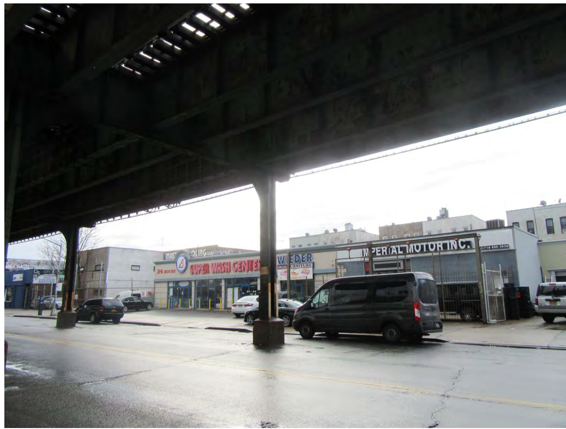
28. View of the side of McDonald Avenue facing southwest between Quentin Road and Woodside Avenue.
