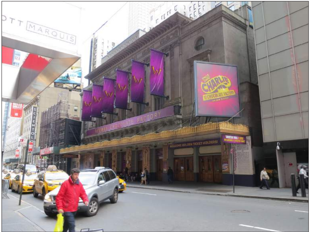
View northwest of the Globe Theater at 203-217 West 46th Street 8
