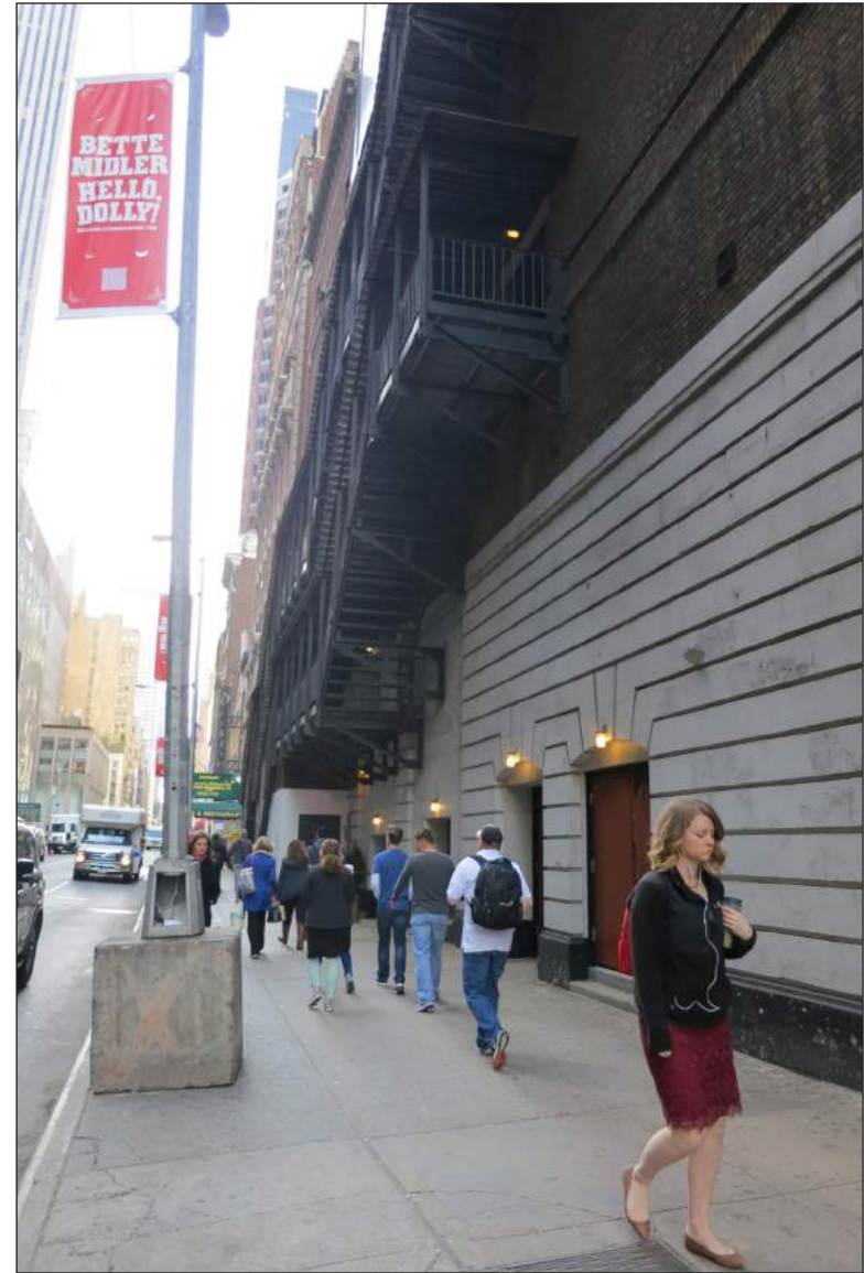
View of the project site with projecting fire stairs from West 47th Street near Seventh Avenue looking east. 2
