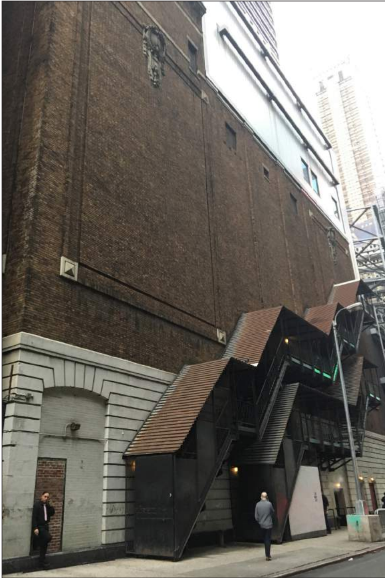
View looking west along 47th Street 1
