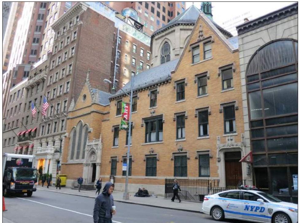
View southeast on West 47th Street of the Church of St. Mary the Virgin lady chapel and rectory
