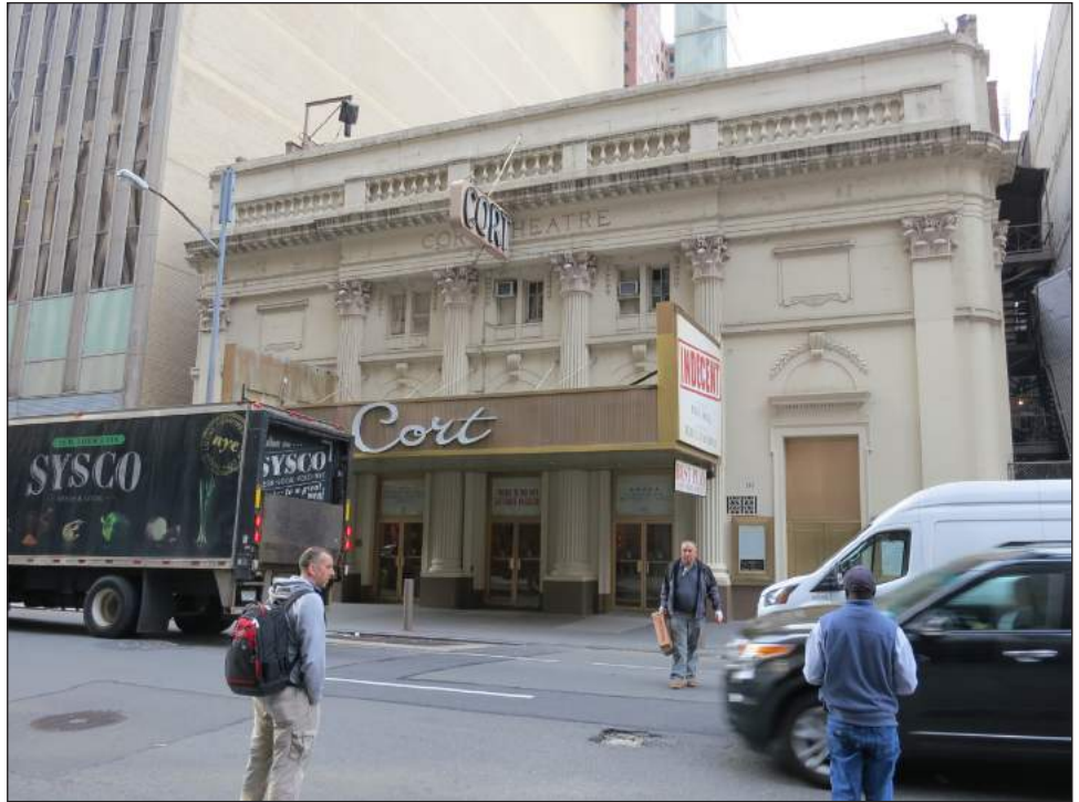
View south of the Cort Theater at 138-146 West 48th Street 9
