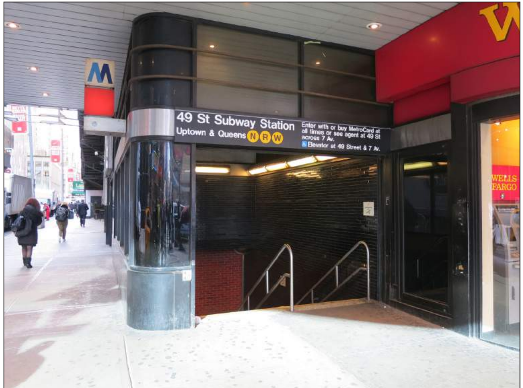
The entrance to the N, R, and W NYCT subway lines is located at the northwest corner of the building. 3
