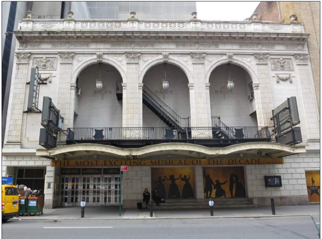
The marquee of the Rogers Theatre and an unenclosed balcony project across the street line. View from West 46th Street between Broadway and Eighth Avenue facing south.
