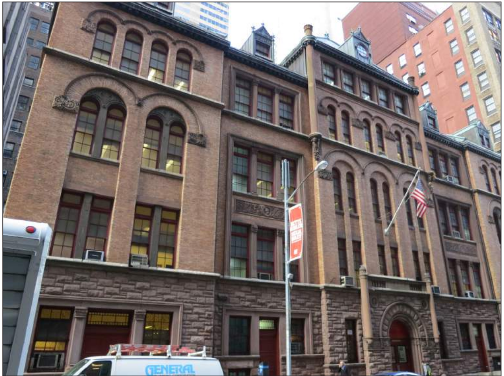
View south of Public School 57 at 120 West 46th Street 6
