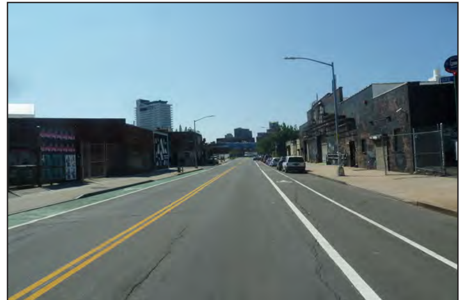
12. Looking south along Franklin Street from the intersection of Quay and Franklin Street
