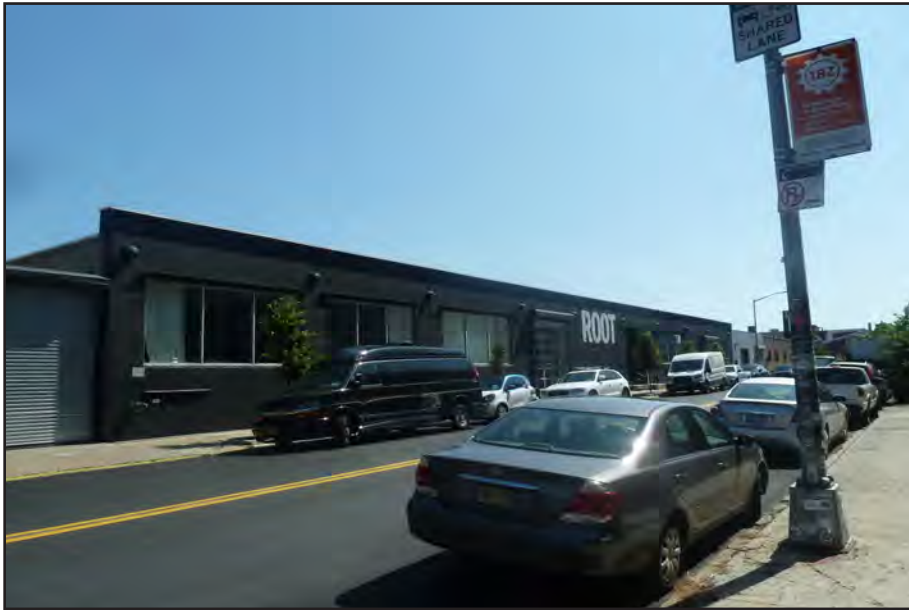
9. Looking east at a converted building on North 14th Street
