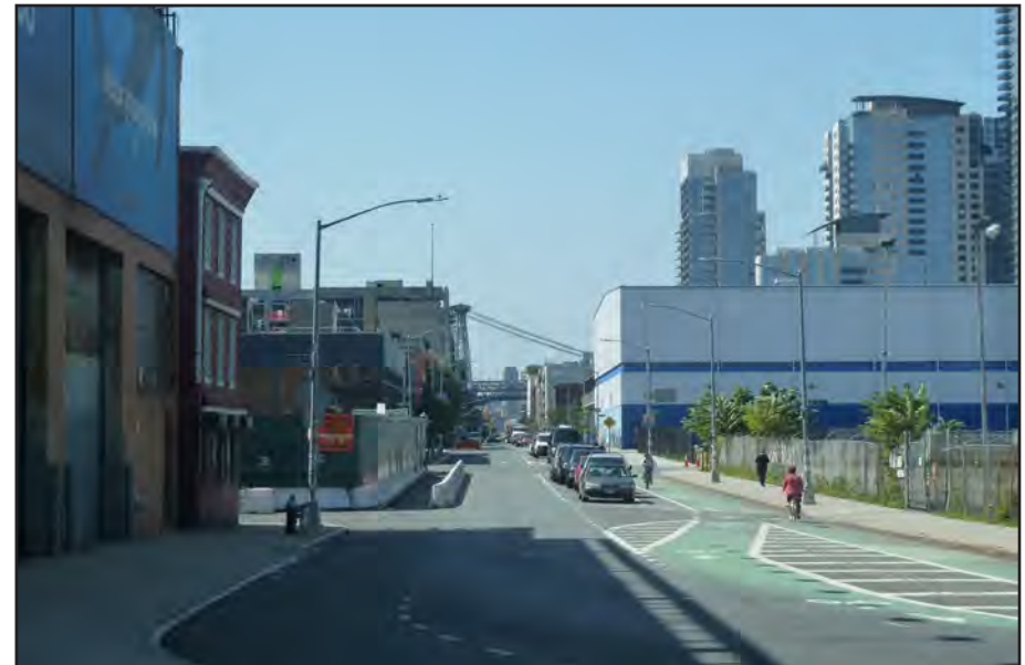
20. Facing south down Kent Avenue at the Williamsburg Bridge
