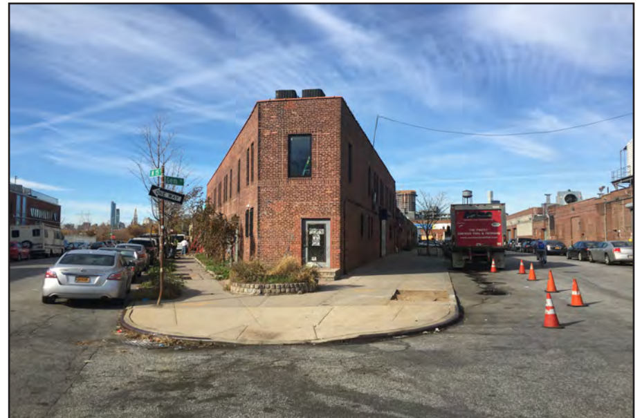
4. Intersection of North 15th Street and Gem Street looking northwest
