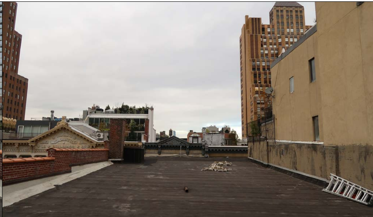
PHOTO 5 - VIEW OF ROOF FROM SOUTH
