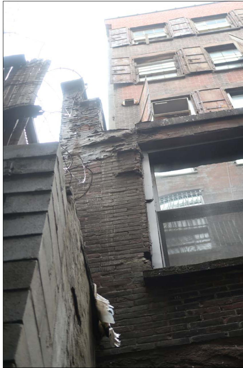
PHOTO 3 - VIEW OF FRONT REAR FACADE FROM COURT
