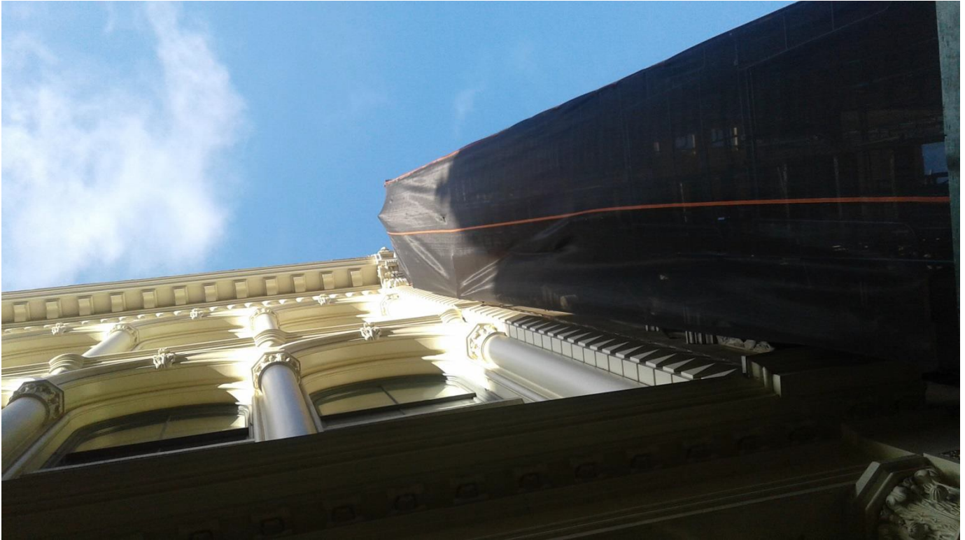
Location 2: Looking up at Location 2 from White Street.
