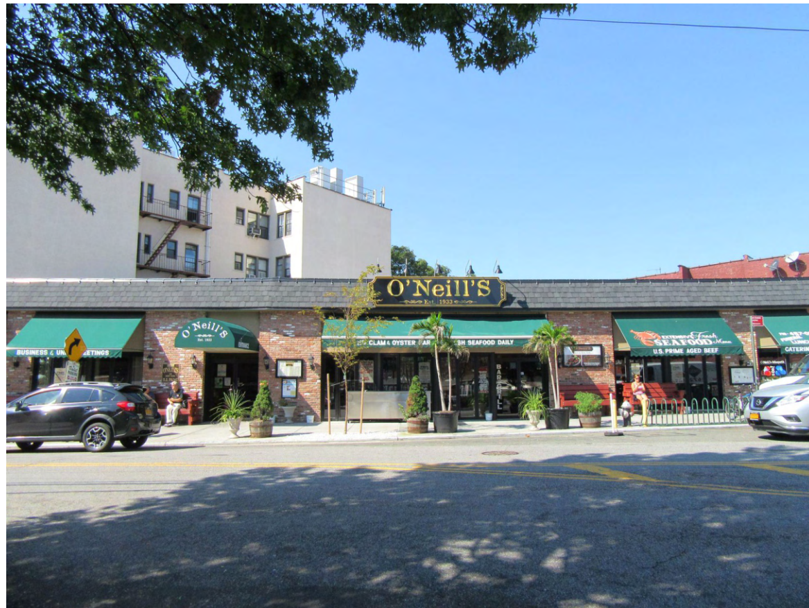
3. View of the Site facing northwest from the intersection of 53rd Drive and 65th Place.
