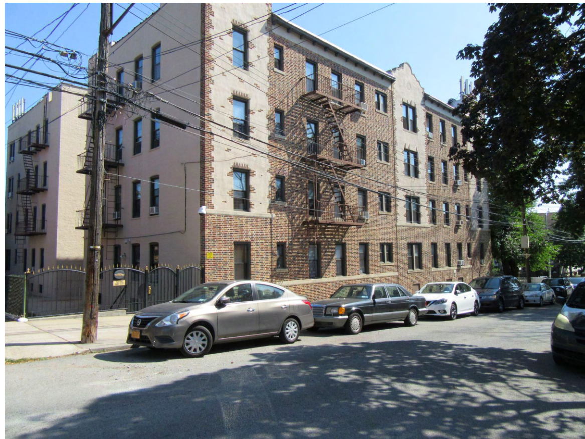
12. View of the Project Area facing southeast from 64th Street.
