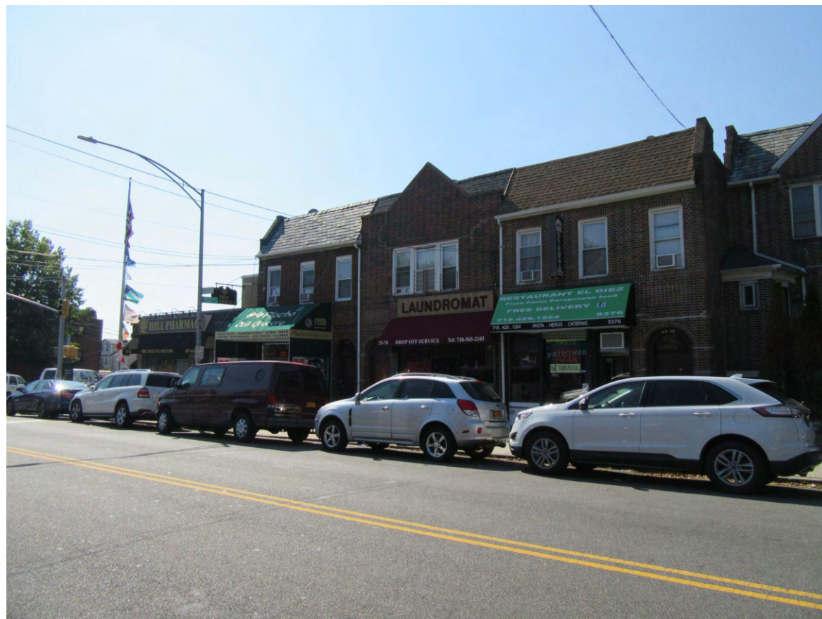
31. View of the Project Area facing southwest from 65th Place.
