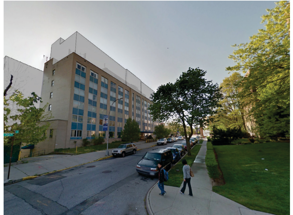
113th Street facing south (Site at left)
