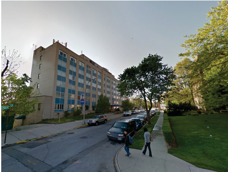
113th Street facing south (Site at left)
