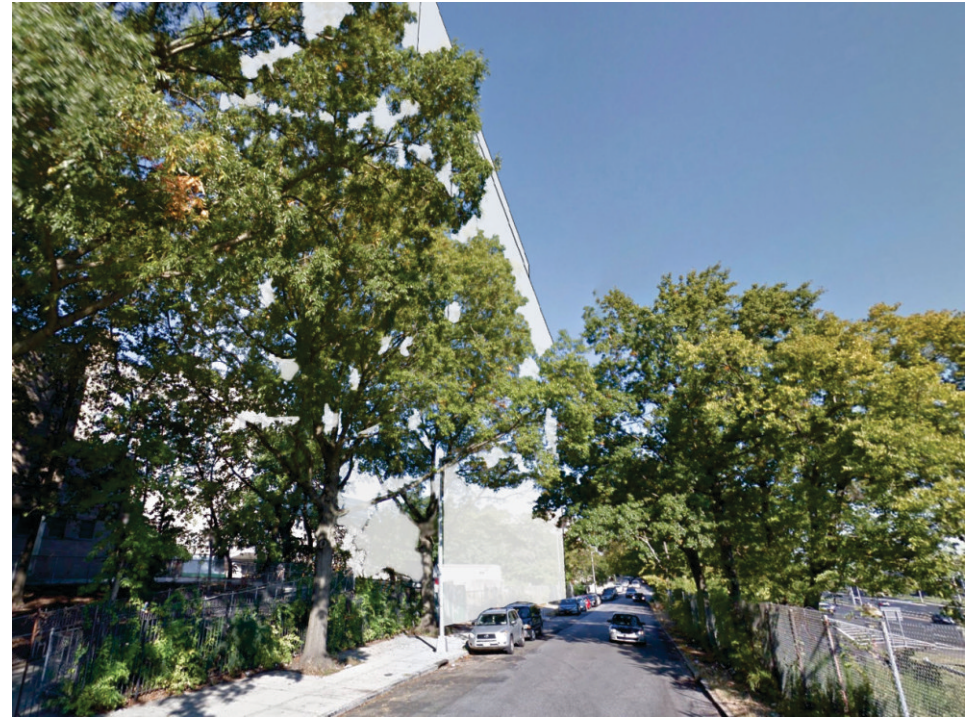
Grand Central Parkway facing north (Site at left)
